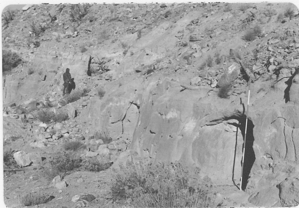
Photo (a) Looking northwestward at two interconnecting adits center and right, and collapse hole, directly in front of person. Hole formed when a drift parallel to the face collapsed. Adits are 5' high x 5' wide; note range pole.
