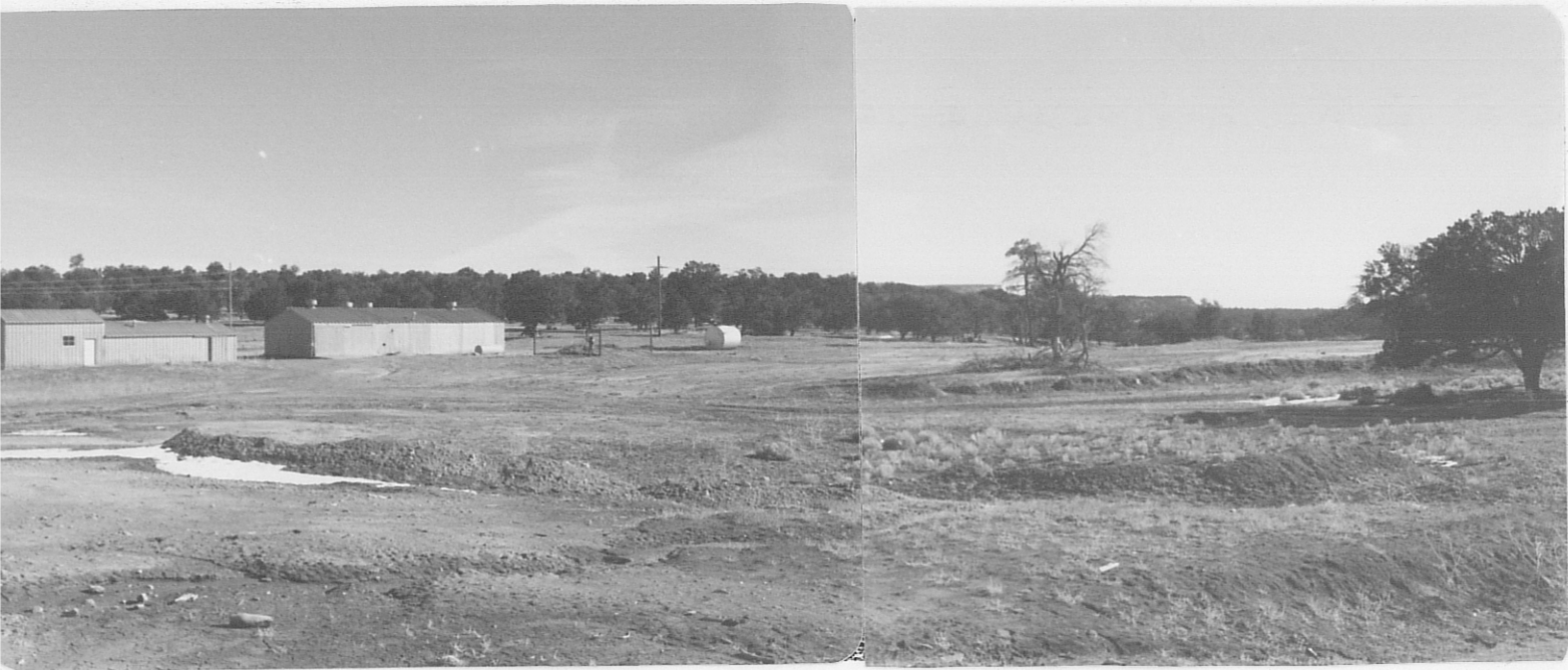
Photo (a) Panorama looking north at the buildings and shaft (circled) at the Mac #1 Mine. The main dump is in the foreground, and the circular dump is on the right center of the photo (as indicated by geologist).
