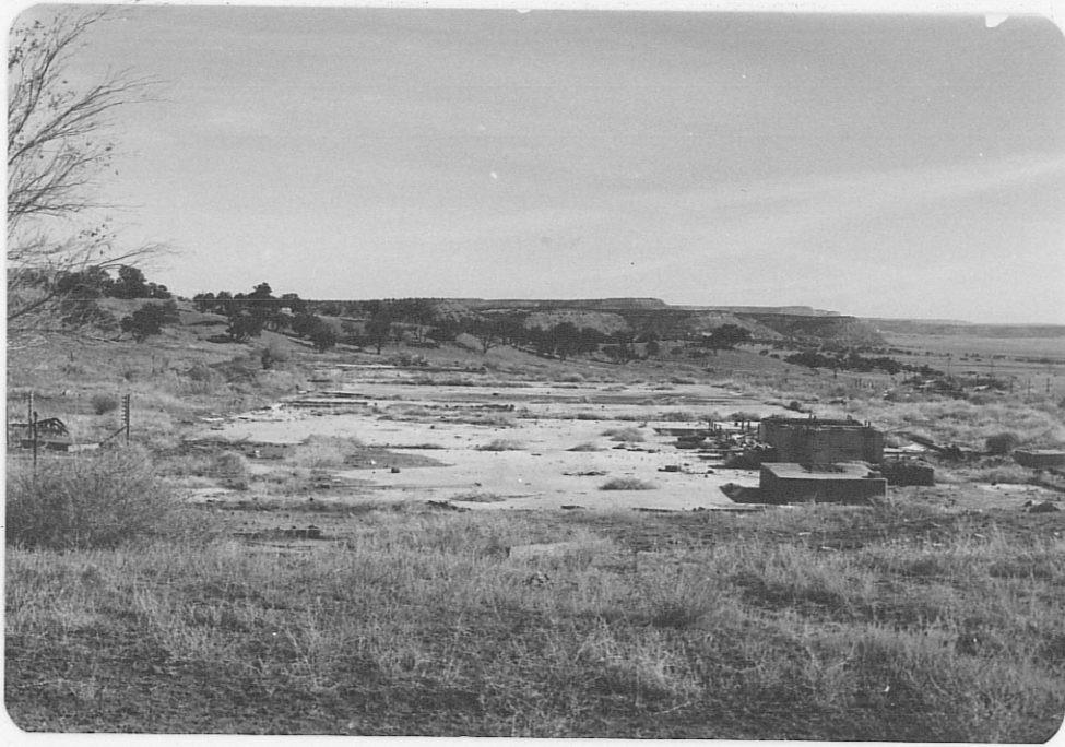
Photo (c) Looking east at 190' long concrete slab; hoist and drum foundation at right.
