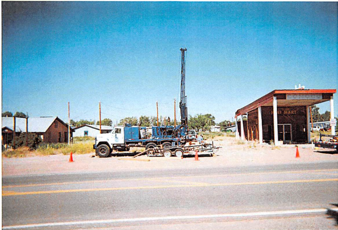
No. 5 – View looking west during the drilling of soil boring SB-7/MW-6.
