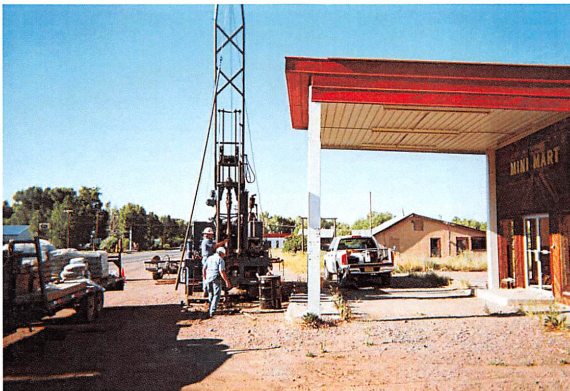
No. 4 – View looking southeast during the drilling of soil boring SB-6/MW-5.
