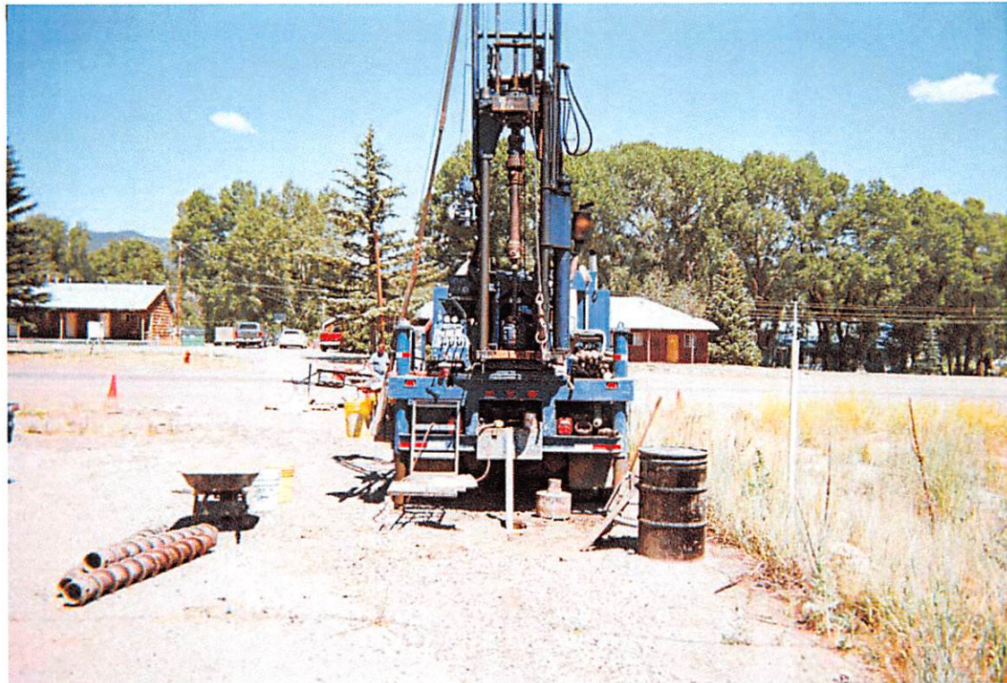
No. 6 – View looking east during the drilling of soil boring SB-8/MW-7.
