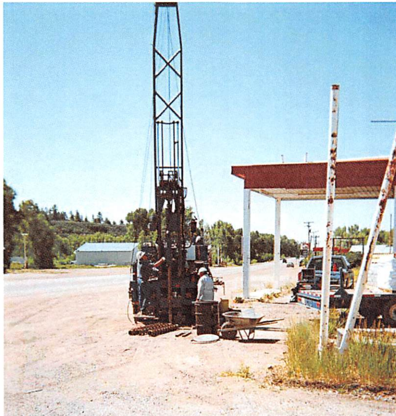
No. 3 – View looking southeast during drilling of soil boring SB-5/MW-4.
