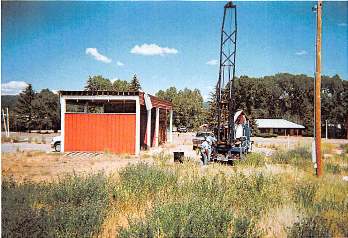
No. 7 – View looking west during the drilling of soil boring SB-9/MW-8.
