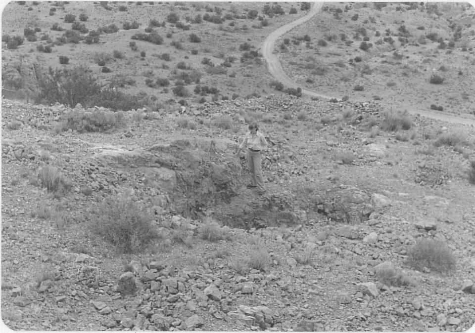
Photo (a) Looking eastward at 8'x 12' open pit on Little Davie workings; access road shows in background. Size of waste pile in background indicates additional stripping in immediate area.
