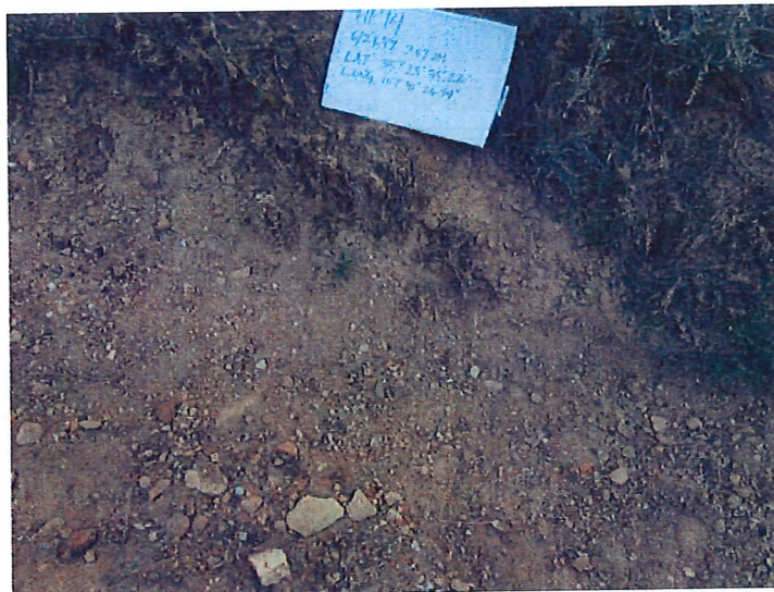
15 - HP14 example of debris at base of channel
