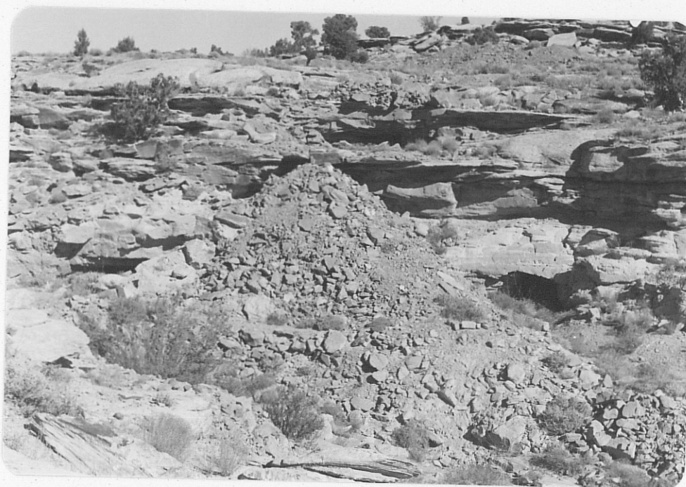
Photo (i) VCA Plot #7, SE side, looking E at two stub adits (upper one partially concealed by tailings from open cut above); on east side of small N-S tributary to Oak Spring Wash. Adit at lower right is approx. 5' high, 6' W, 12' long; see also photo (j).
