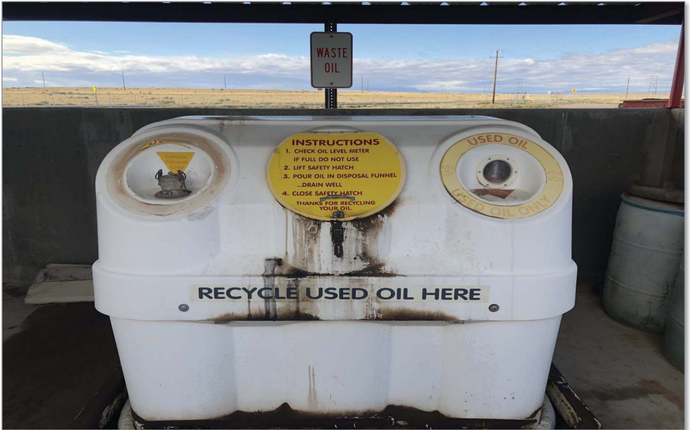
FIGURE 1-5: WASTE OIL SIGN: DISPOSAL/HOLDING AREA
