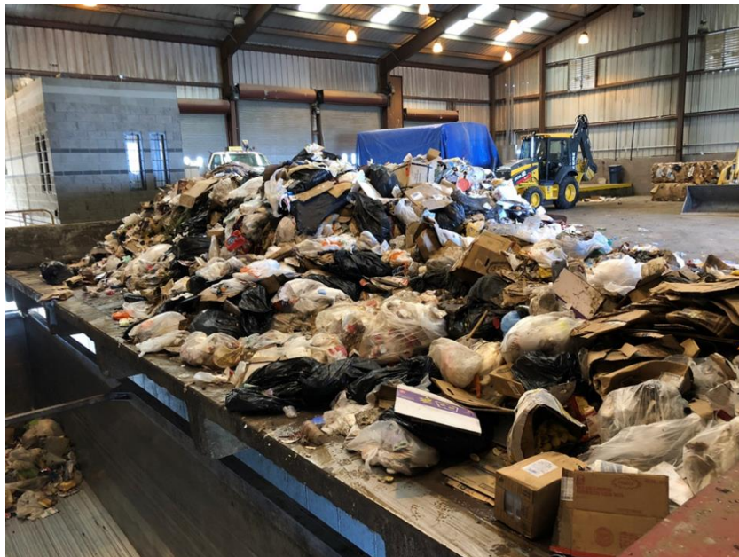
FIGURE 6-2 UPPER LEVEL OF TIPPING FLOOR WITH LEDGE ABOVE OPENING OF THE COLLECTION TRUCK
