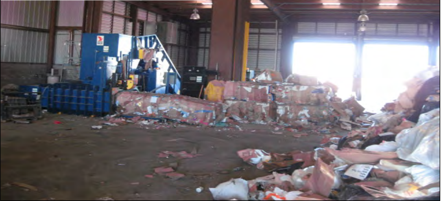
3/14/2017, 2:19 PM, #001 Los Lunas Transfer Station Photographer: Paul E. Martinez, NMED/SWB View of tipping floor near bale facility operation. Facing W
