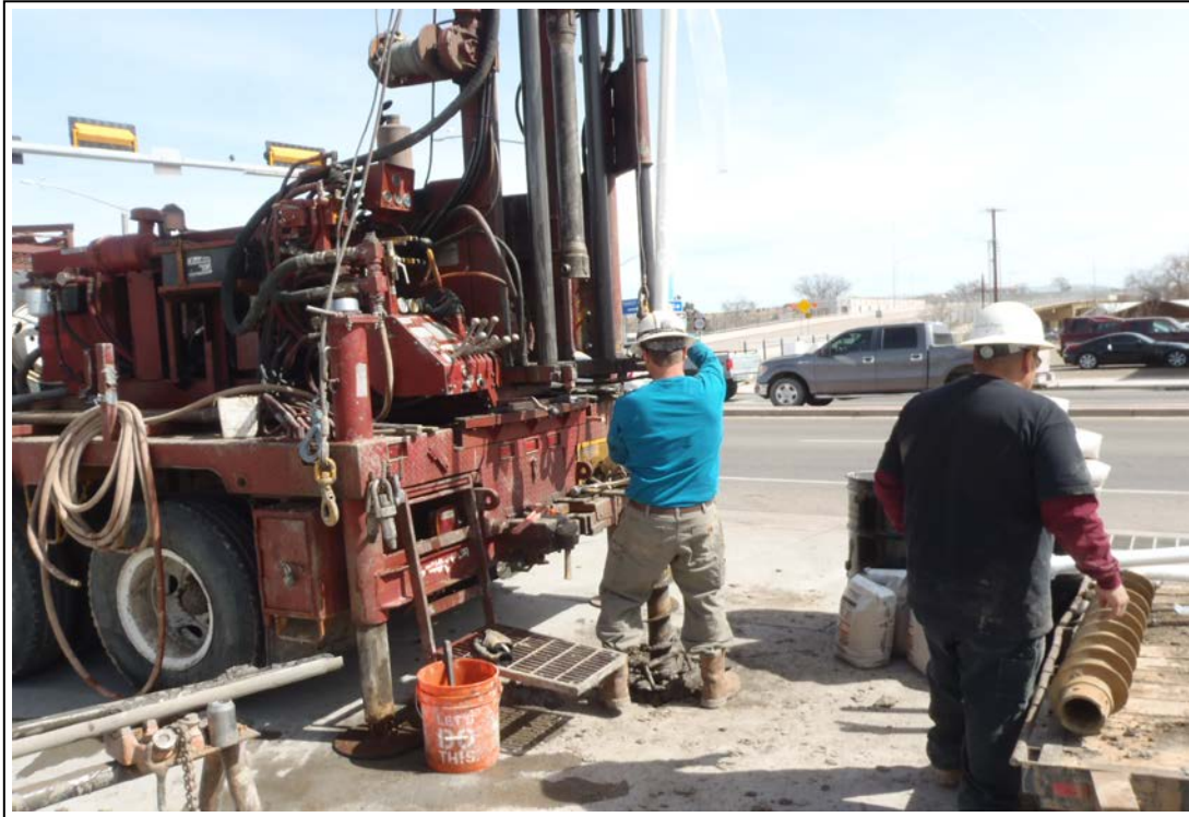
1. Drilling monitor well MWAL-2R (view to the east)
