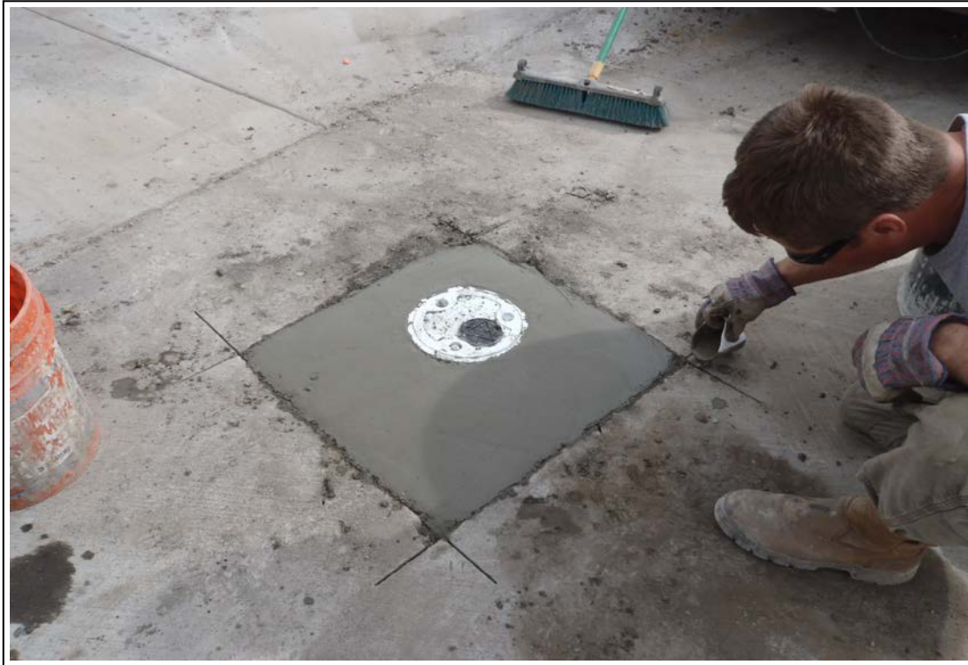
5. Monitor well MWAL-2R well pad installed (view to the southeast)
