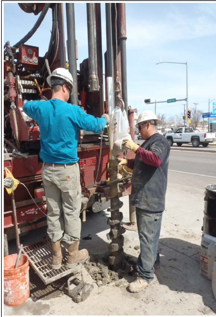
3. Installing filter pack during monitor well MWAL-2R construction (view to the northeast)
