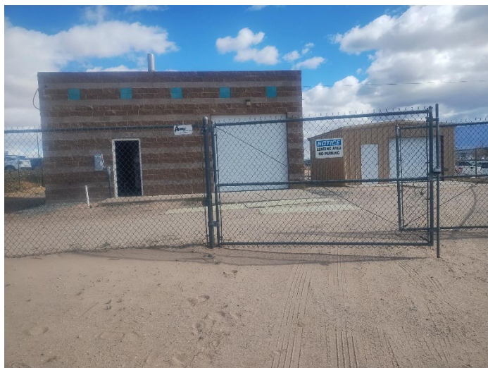
CW-2 Pump house and storage building
