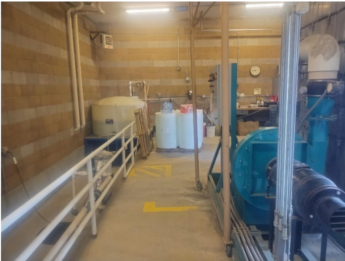
CW-2 Aquamag tank, sump and air stripper
