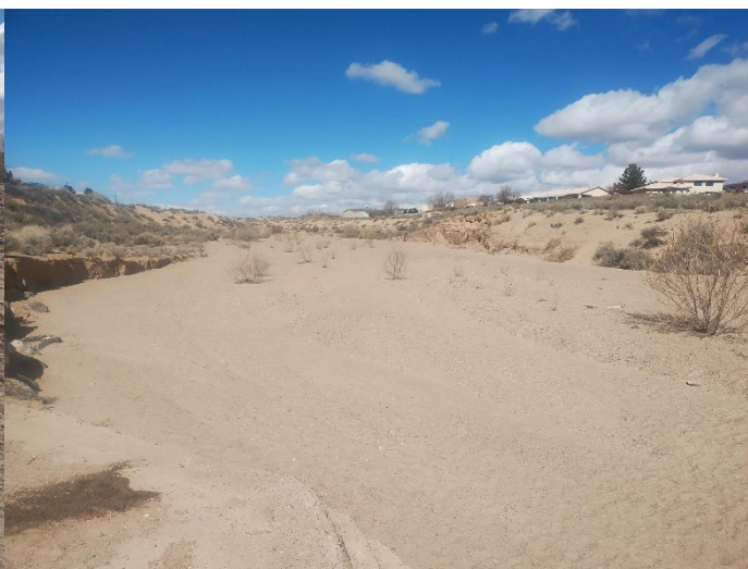
CW-1 Infiltration Gallery looking West
