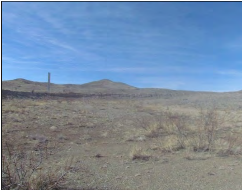
Figure 3-30. View of Tailing Pond and Tower
