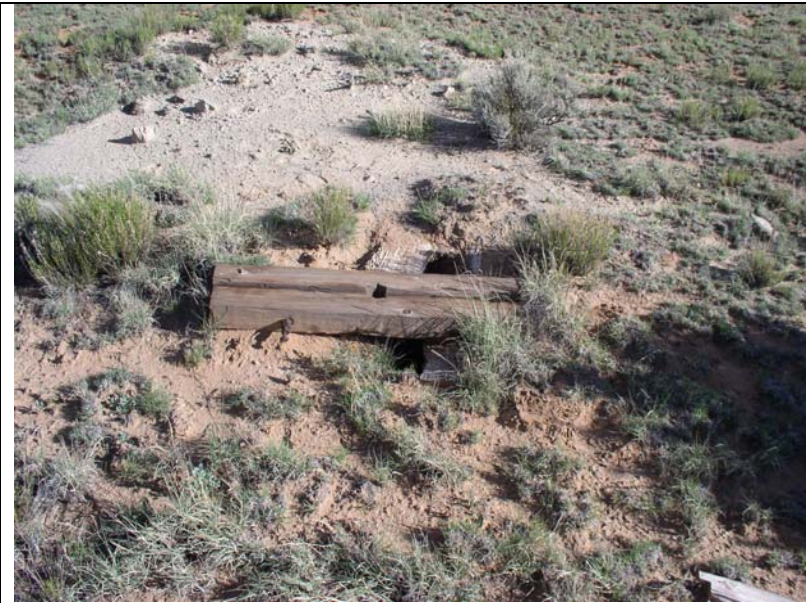
P3: Blue Peak mine open vent shaft on mesa top.
