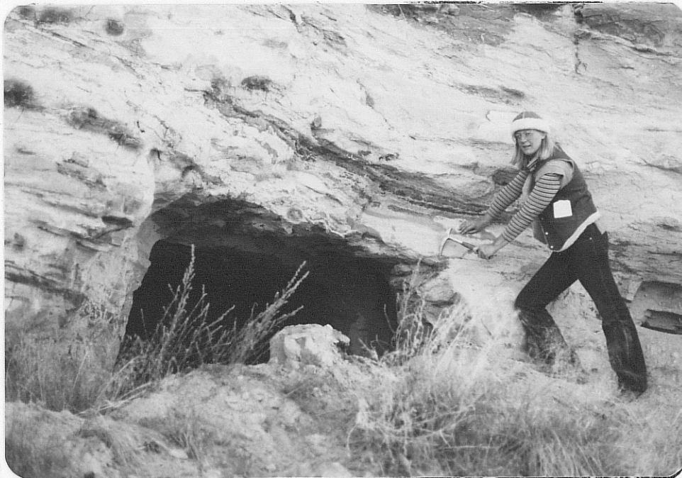
Photo (c) Key and Tohe workings; powder magazine to left of main adit.
