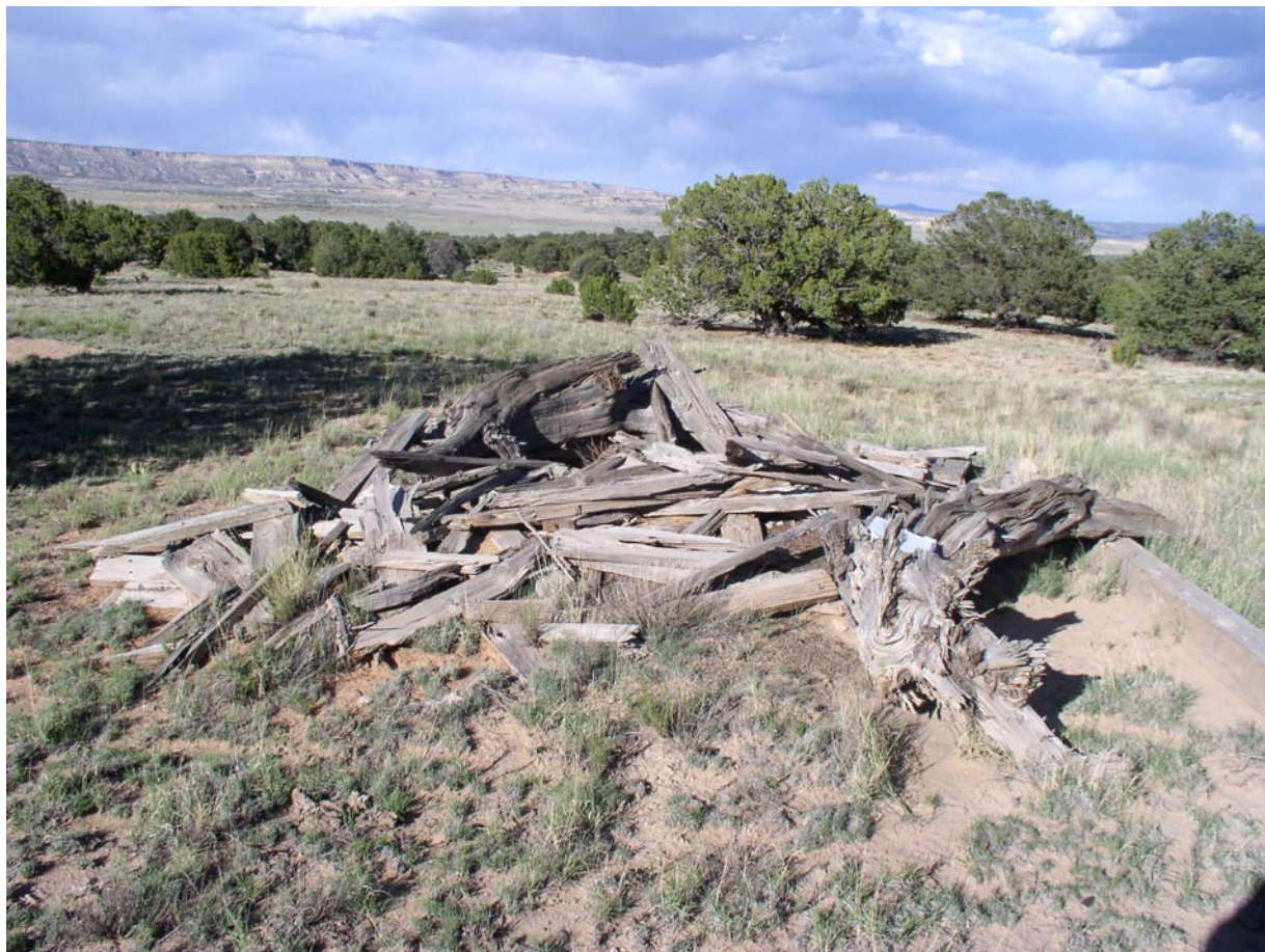
P1: Davenport Mine collapsed frame structure
