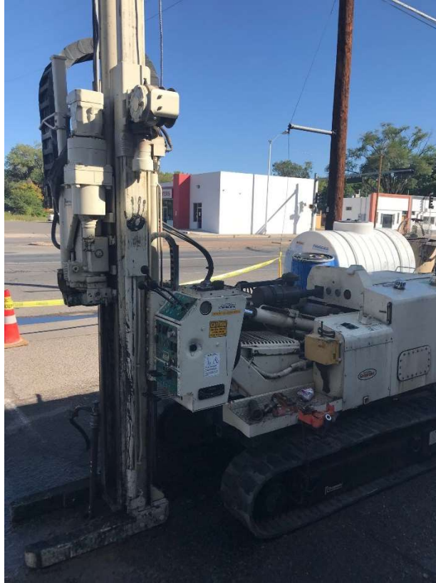
GeoProbe® 7720DT Rig Used to Inject PetroFix®
