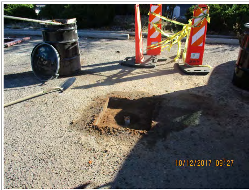
13. Asphalt cut-out for monitor well MW-18.
