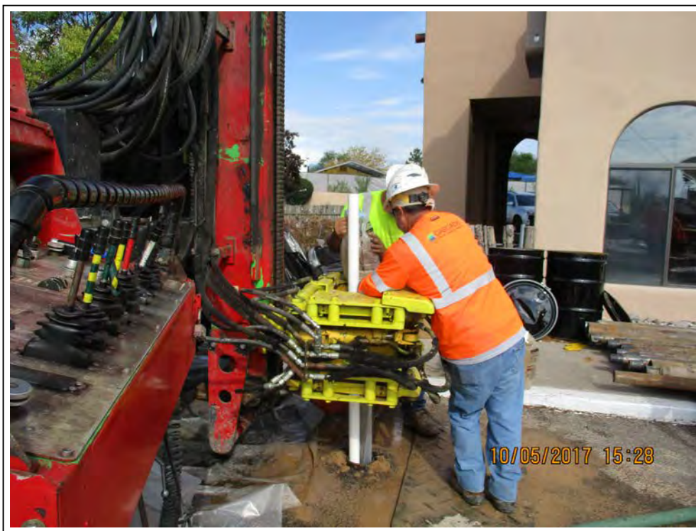
6. Installing monitor well MW-16.
