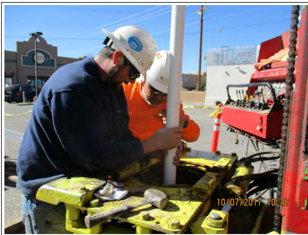
12. Installing monitor well MW-18.
