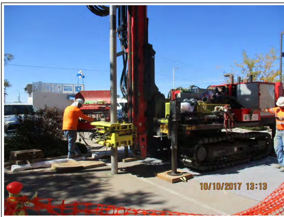
14. Set up to drill borehole MW-19, view to the southwest.
