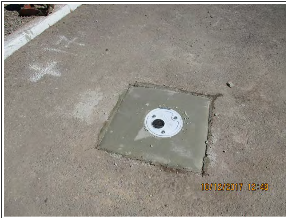
10. Monitor well MW-17 surface completion.
