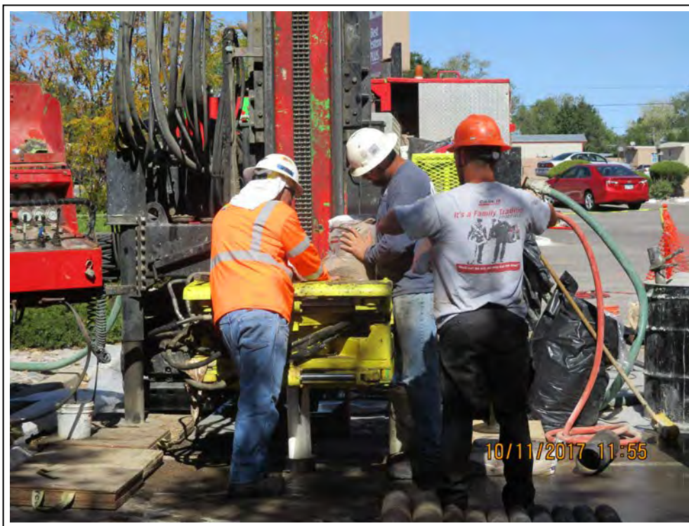
15. Installing sand filter pack at monitor well MW-19.
