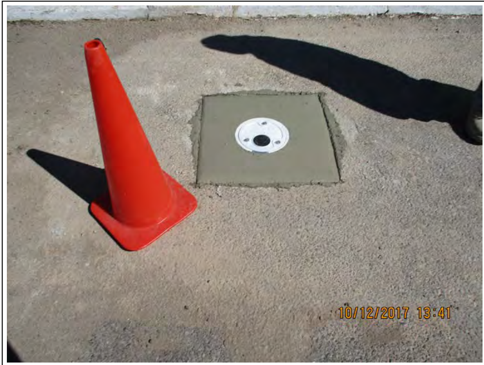
7. Monitor well MW-16 surface completion.
