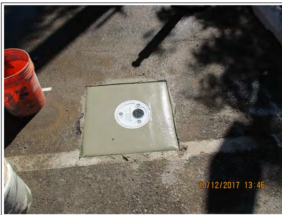
16. Monitor well MW-19 surface completion.
