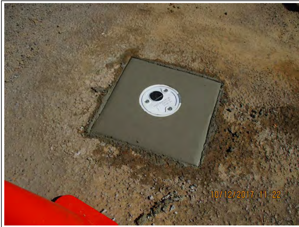
3. Monitor well MW-15 surface completion.
