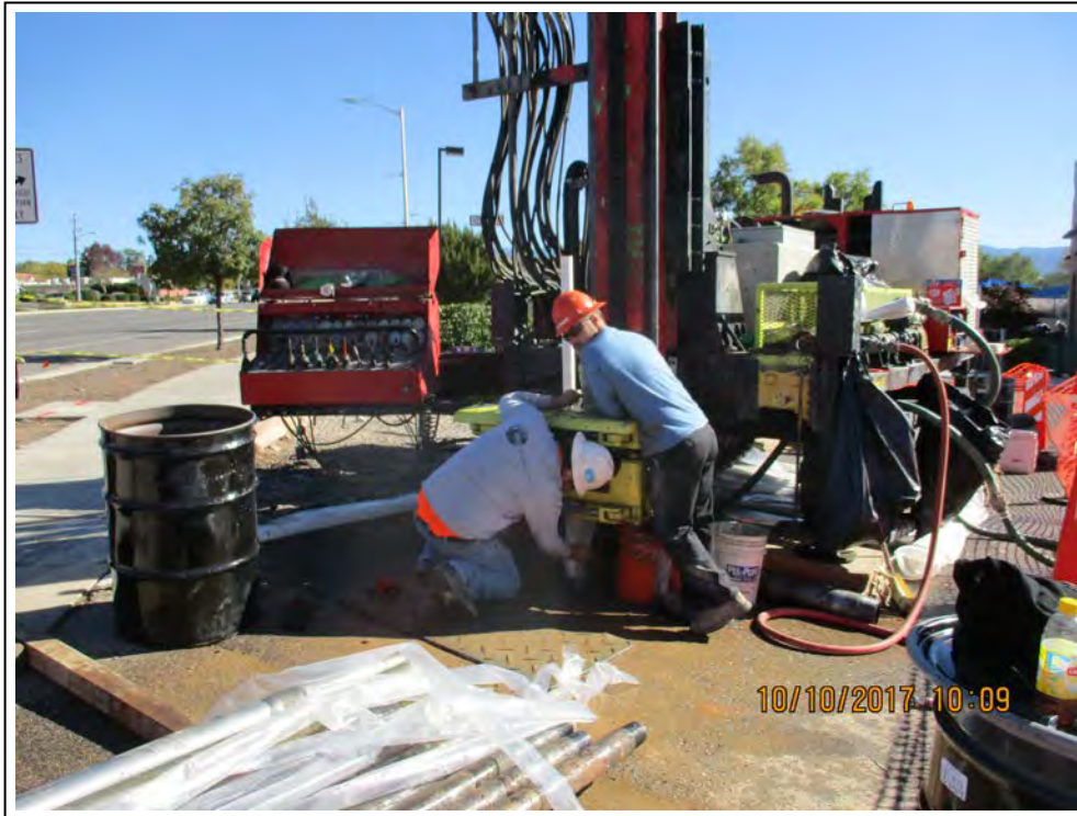
9. Installing monitor well MW-17 well casing, view to the northeast.
