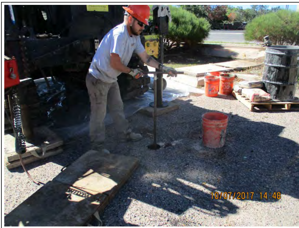
1. Potholing to check for utilities at borehole MW-15.
