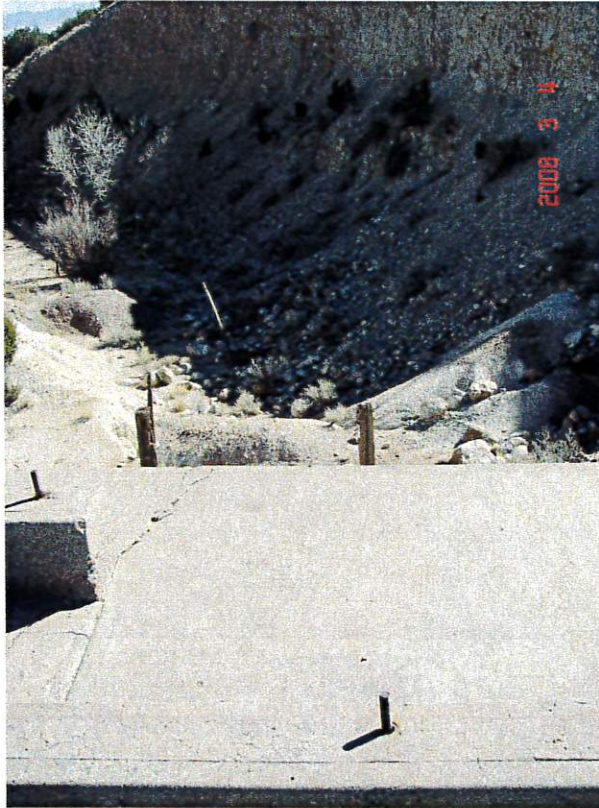
View east into cut from pad
