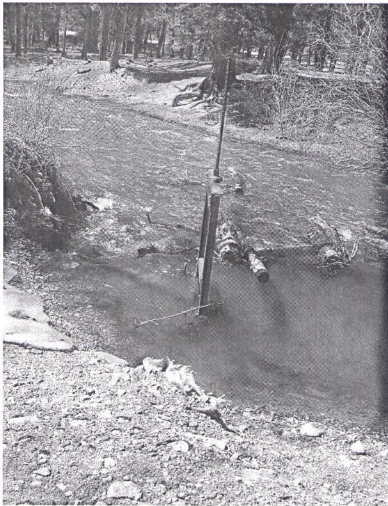
Existing headgate at Fawn Lakes
