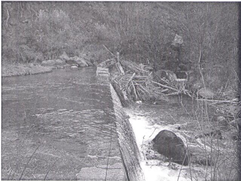
The hatchery diversion structure, an effective migration barrier
