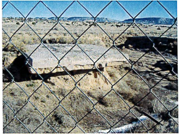
Pad, arroyo, erosion through site
