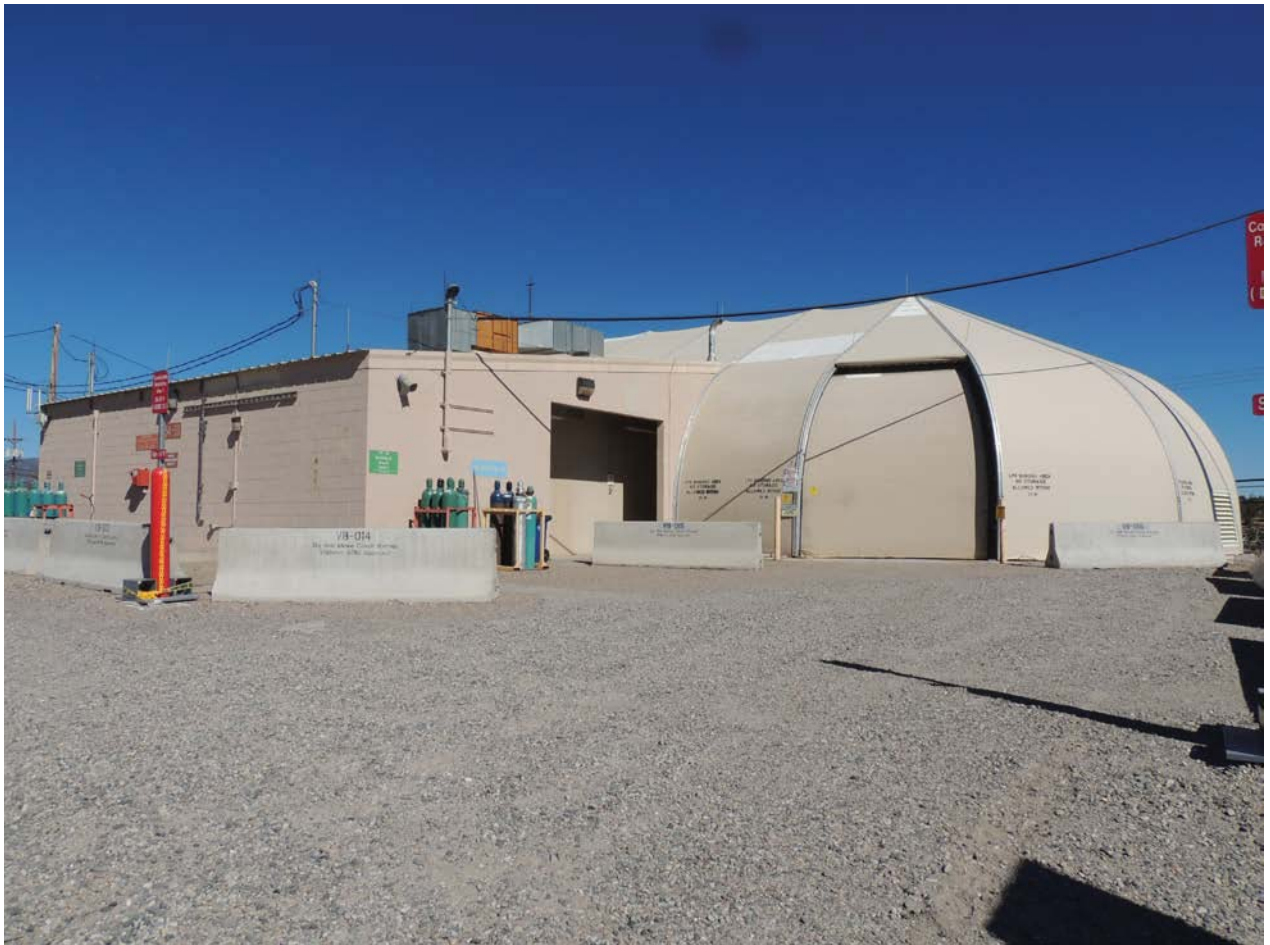
TA-54-33, Area G, Drum Prep Facility Process Code S01, Container Storage Unit
