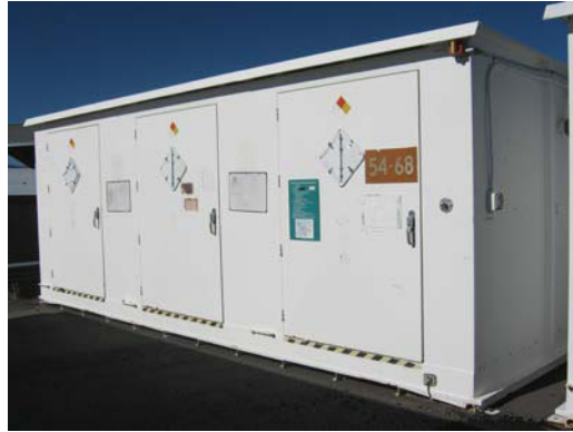
TA-54-68, Area L, Process Code S01, Container Storage (Modular Storage Building 68)
