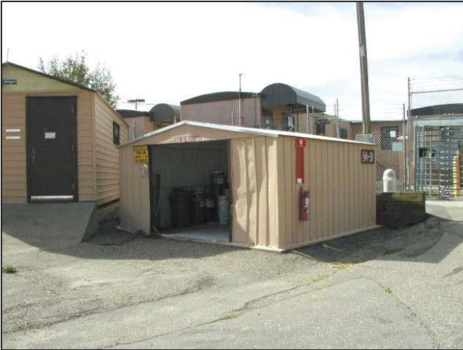
TA-54-31, Area L, Process Code S01, Container Storage Unit
