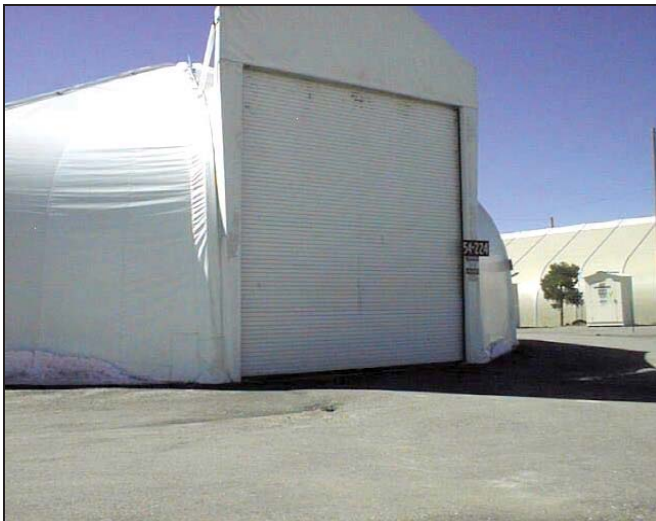
TA-54-224, Area G, Storage Dome Process Code S01, Container Storage (Consolidated Pad No. 5, Formerly Pad Nos. 5, 7, and 8)
