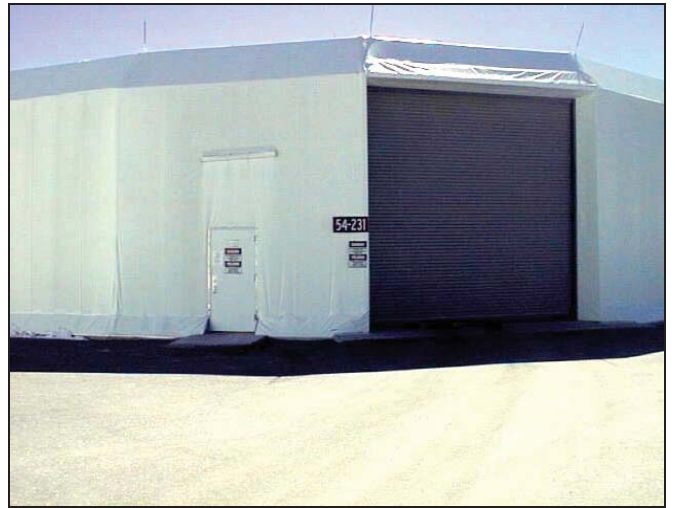
TA-54-231, Area G, Storage Dome Process Code S01, Container Storage (Pad No. 9)
