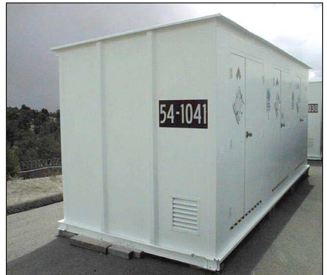
TA-54-1041, Area G, Storage Shed Process Code S01, Container Storage (Consolidated Pad No. 5, Formerly Pad Nos. 5, 7, and 8)
