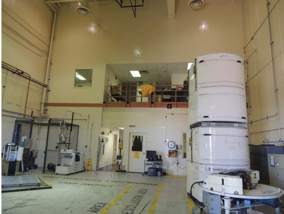
TA-54-38 West Indoor, Low Bay, Process Code S01, Container Storage Unit
