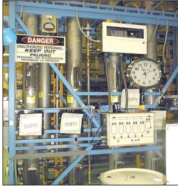
TA-55-4, Room 401, Stabilization Unit Pencil Tanks Component, Process Code S02, Storage Tank System
