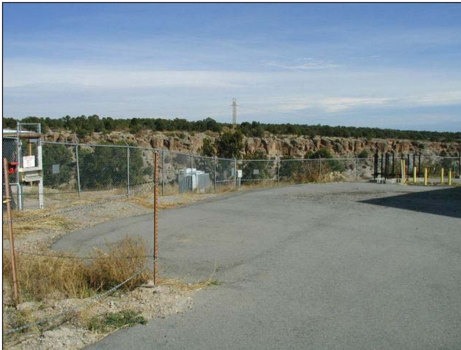
TA-54, Area L, Process Code D80, Disposal Shafts 29-34 (To be closed)
