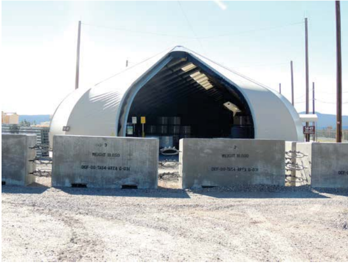
TA-54-49, Area G, Storage Dome, Process Code S01, Container Storage (Consolidated Pad No. 5, Formerly Pad Nos. 5, 7, and 8)
