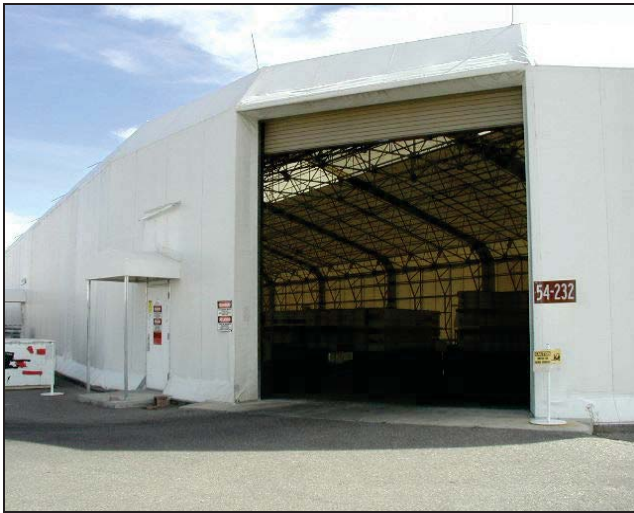
TA-54-232, Area G, Storage Dome Process Code S01, Container Storage (Pad No. 9)
