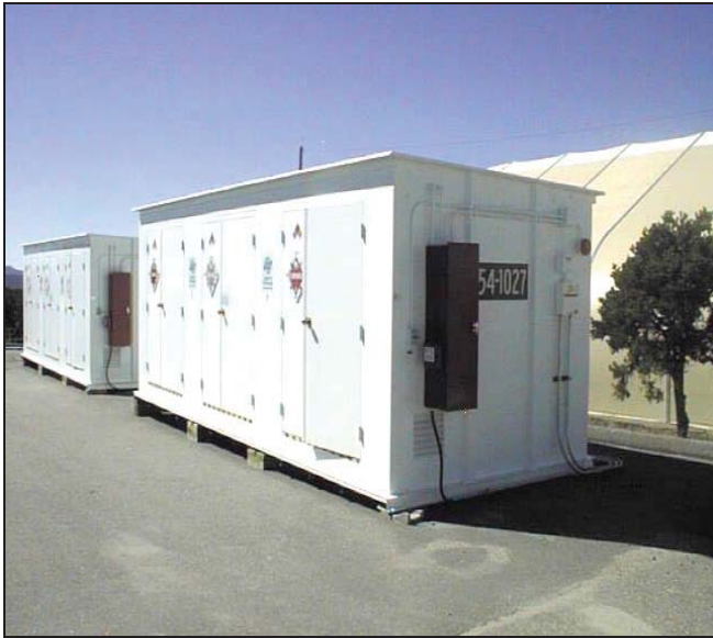
TA-54-1027, Area G, Pad No. 5, Storage Shed Process Code S01, Container Storage (Consolidated Pad No. 5, Formerly Pad Nos. 5, 7, and 8)
