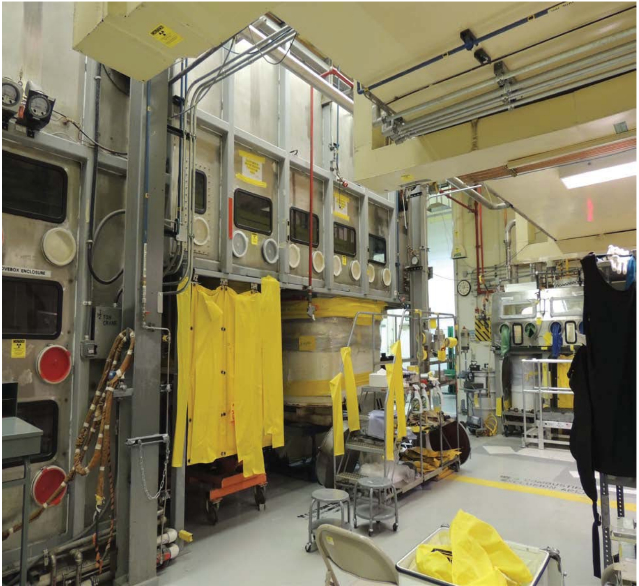
TA-50-69 Indoor, Rooms 102 and 103, Process Code S01, Container Storage Unit
