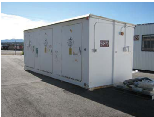
TA-54-70, Area L, Process Code S01, Container Storage (Modular Storage Building 70)
