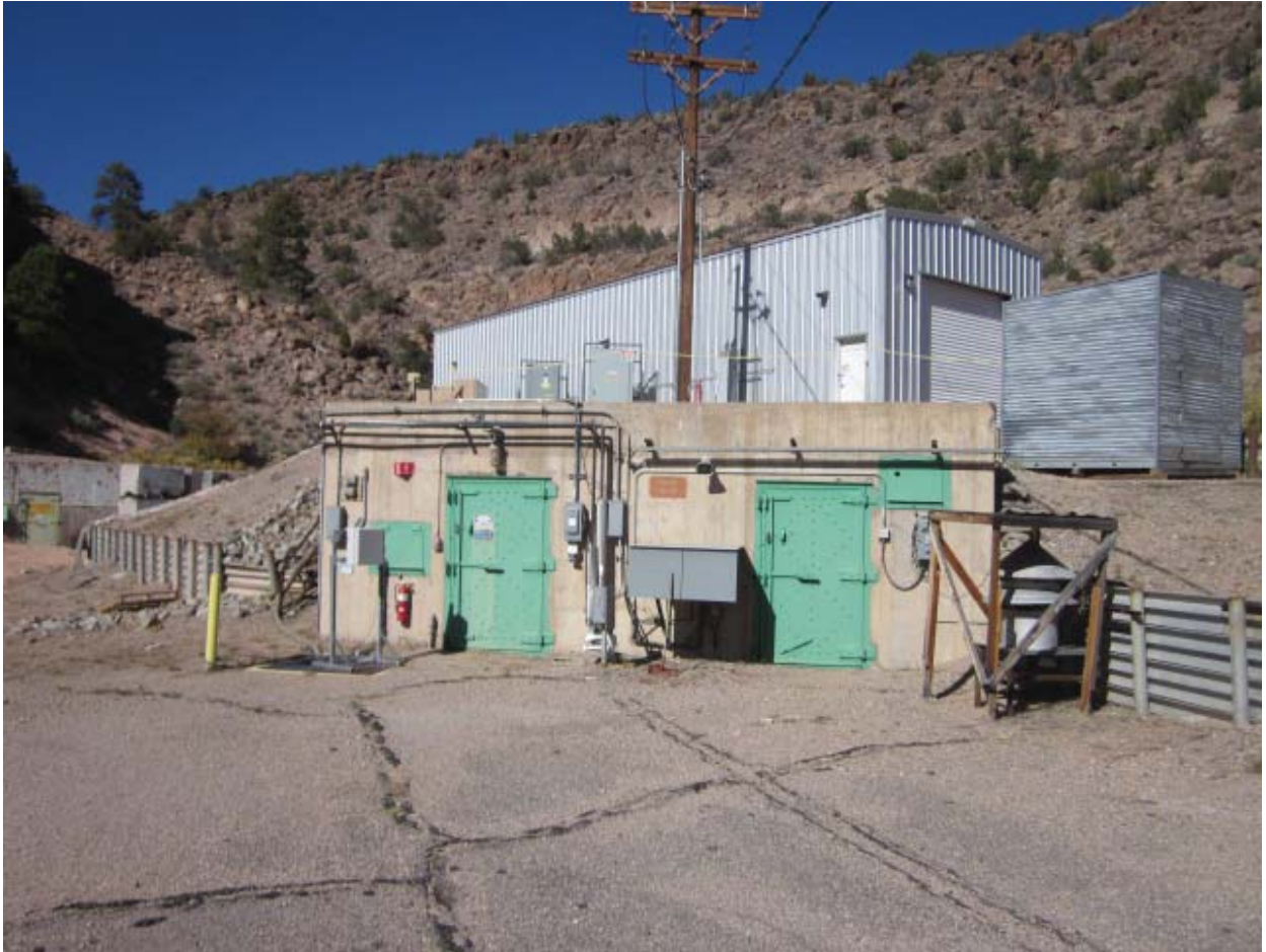
TA-39-57, Process Code X01, Open Detonation Unit
