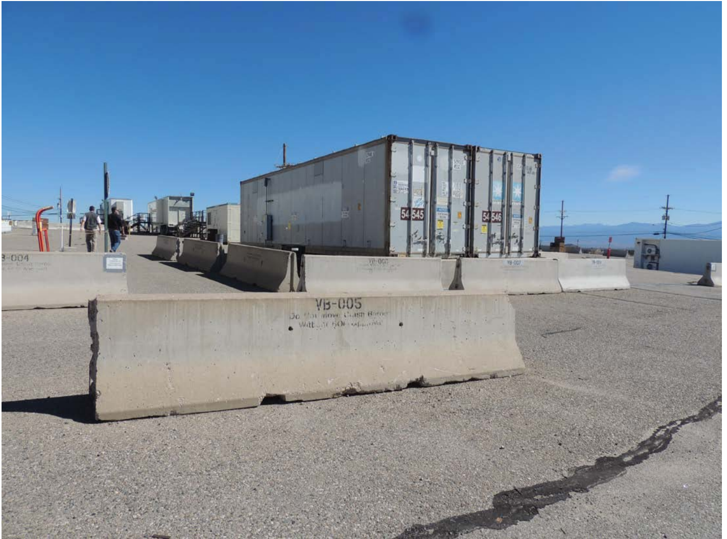
TA-54, Area G, Process Code S01, Container Storage Pad No. 10
