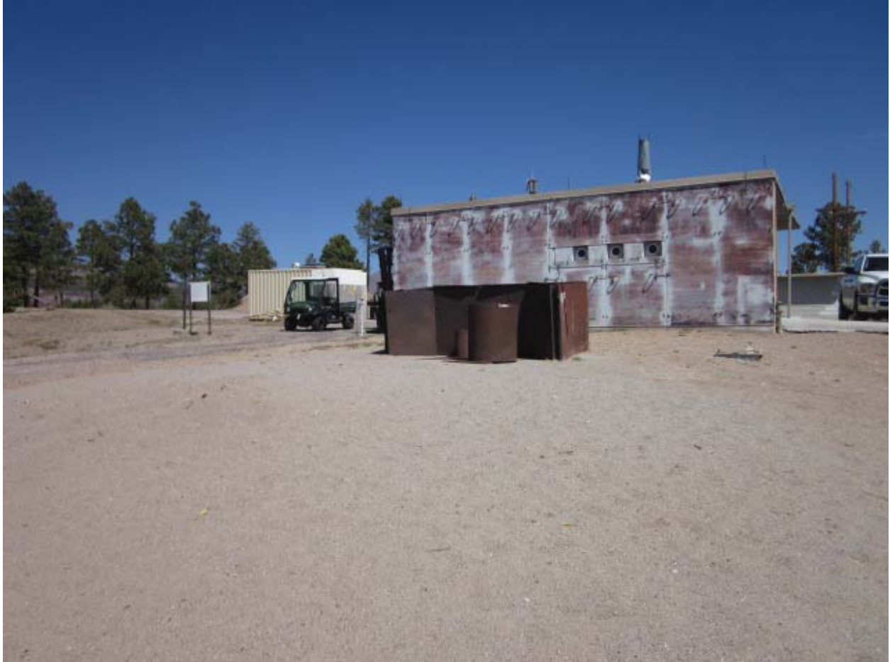
TA-14-23, Process Code X01, Open Detonation Unit (View looking north towards structure TA-14-23)
