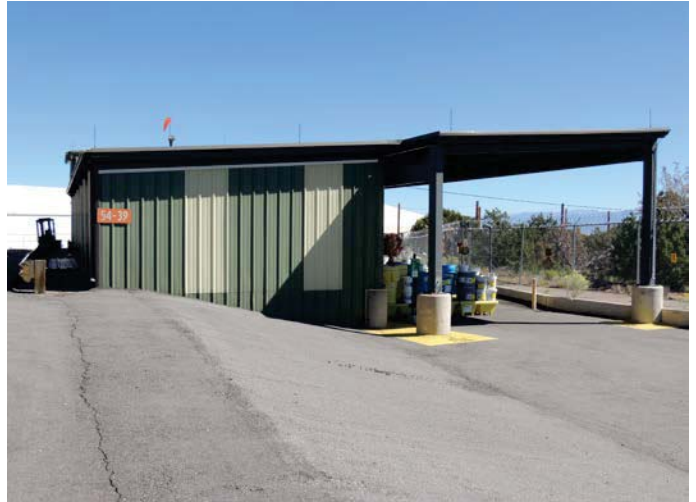
TA-54-39, Area L, Process Code S01, Container Storage Unit
