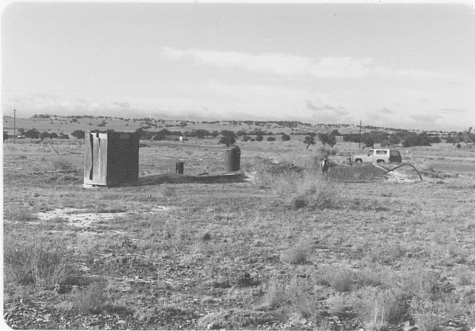
Photo A Looking southwest toward mine shaft site; shaft has been backfilled; note 30" diameter metal ventilation shaft just left of center with 10" diameter pipe left of it, and metal shed at far left.
