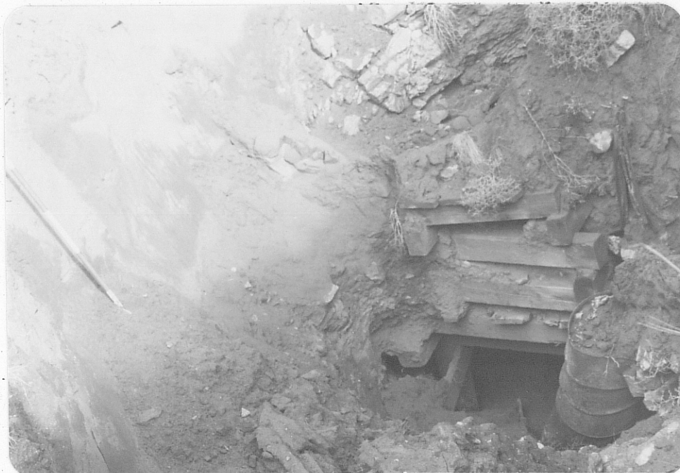
Photo (f) Caved vertical shaft 20' west of decline; hole is presently 22' deep. Note portion of range pole at left for scale.
