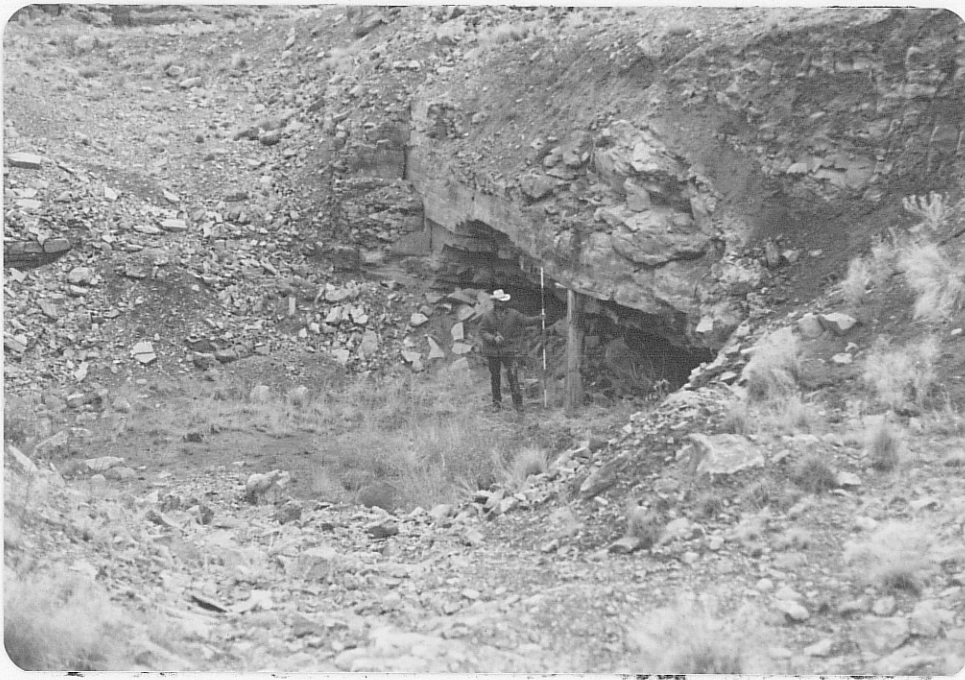
Photo (a) Looking NW at 35' deep pit with some "gophering" along the north face; site is just east of sec. 25-26 line. Scintillometer readings ranged up to 1,100 cps.
