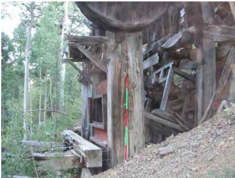
Photo 4-Looking north at StrucPly-1, the stamp mill in Anderson photo A.
