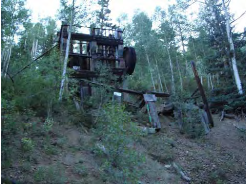
Photo 3-Looking east from Rd-1 at StrucPly-1, the stamp mill in Anderson photo A.
