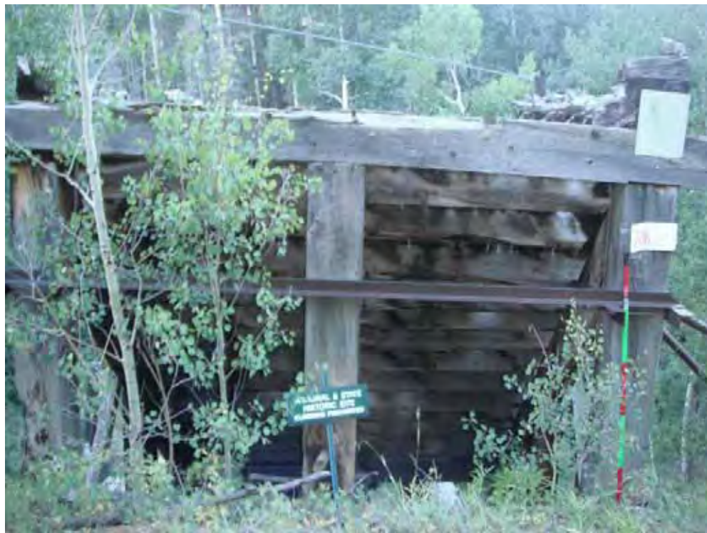
Photo 2-Looking west from Rd-2 at StrucPly-1, the stamp mill in Anderson photo A.
