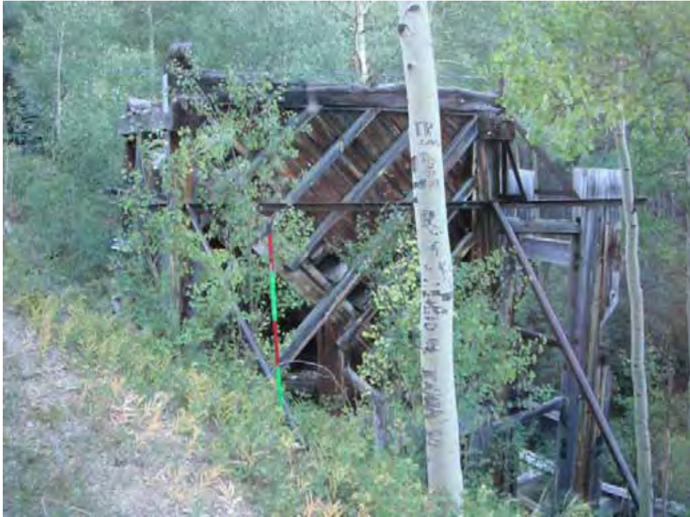
Photo 1-Looking south at StrucPly-1, the stamp mill in Anderson photo A.
