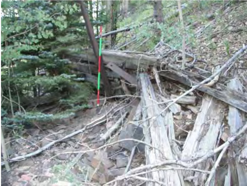
Photo 13-Looking north at StrucLn-1.
