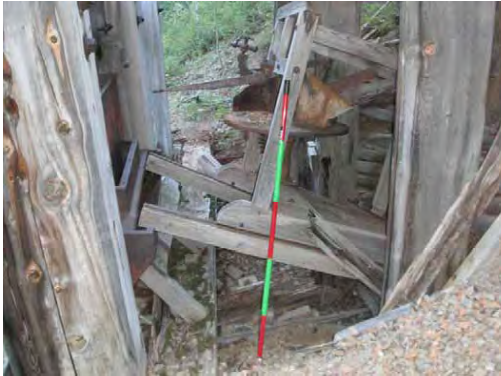
Photo 5-Looking north at StrucPly-1, the stamp mill in Anderson photo A.
