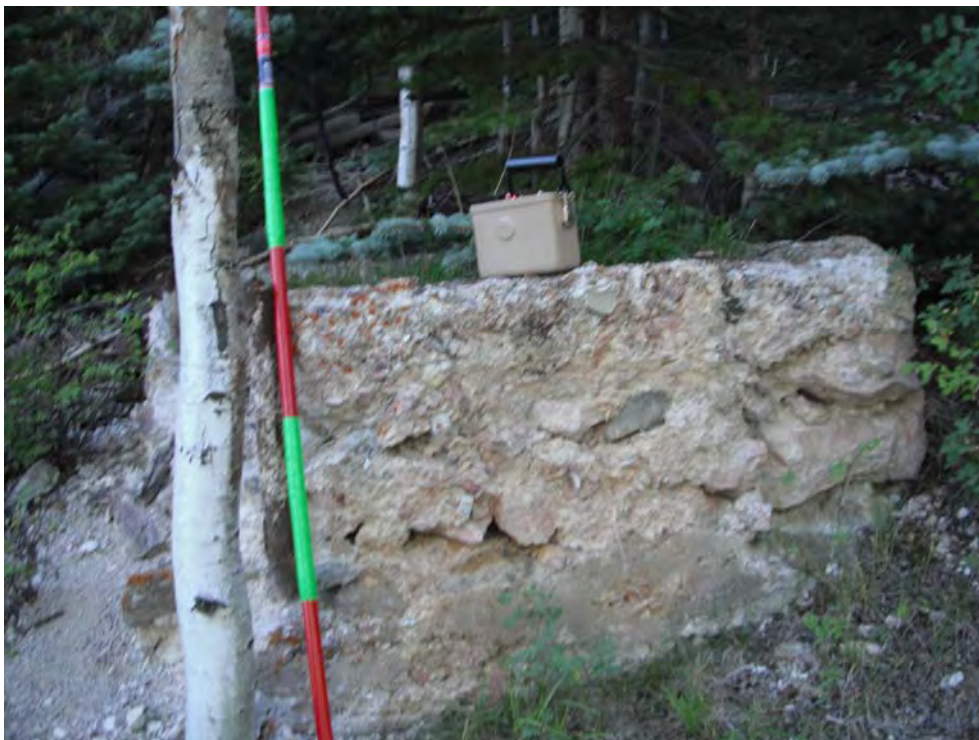
Photo 14-Looking east at StrucPly-3.
