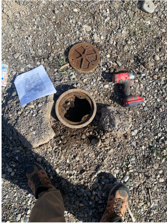
MW-8 vault was in poor condition
