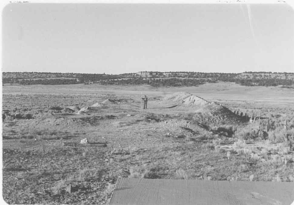
Photo (b) Looking northward from concrete pad in the foreground to the tailings dump. Maximum scintillometer reading on dump was 1,100 cps. Fence on right side of the dump follows the section line.
