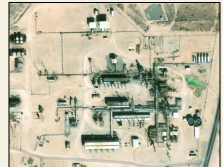
Gas Processing Plant
