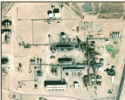
Gas Processing Plant
