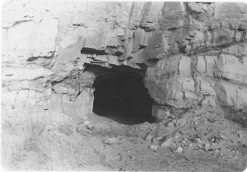
— Photo (c) Looking eastward into 7'x 9' portal of Sec. 8 adit; note field glasses hanging at left of portal for scale.
