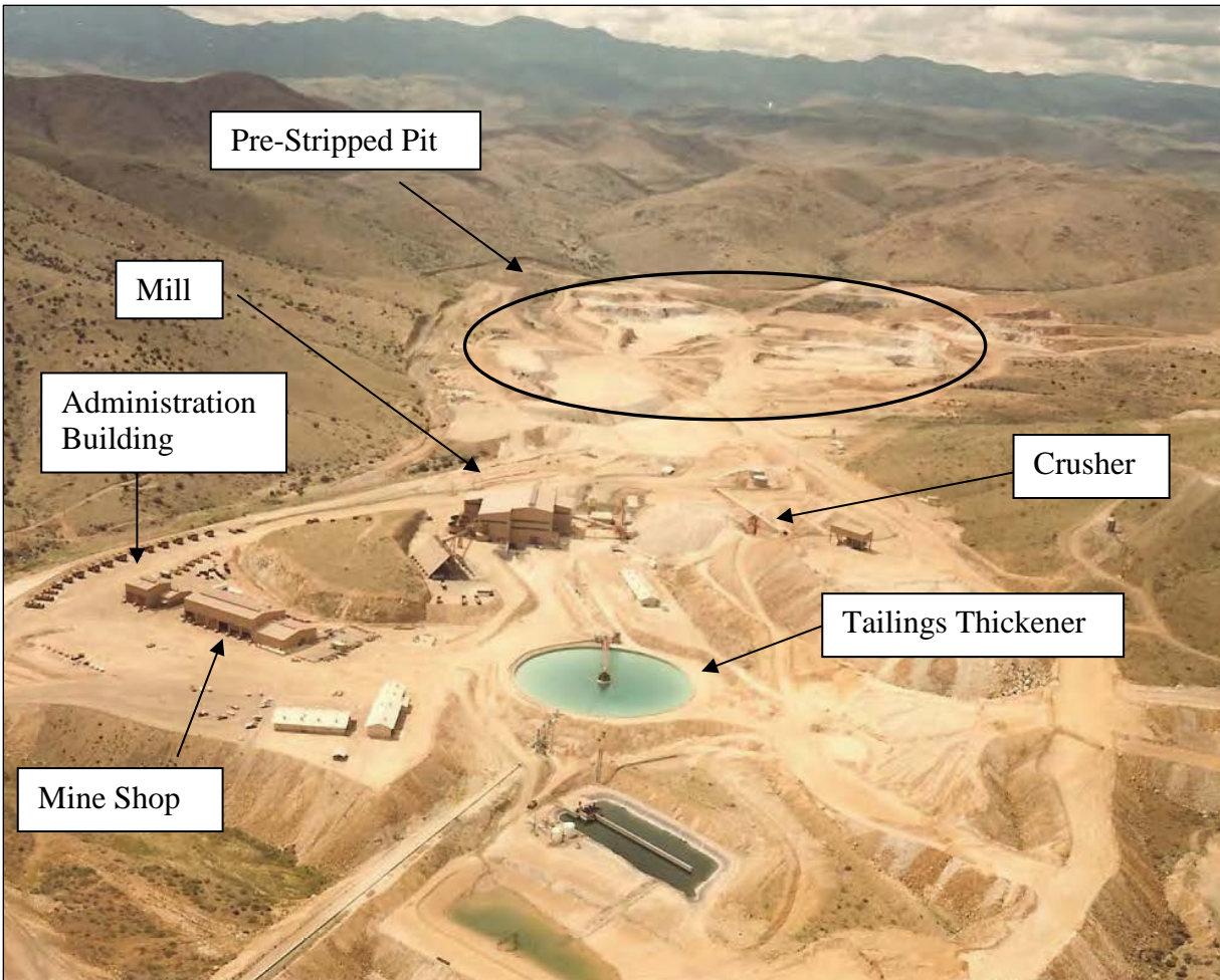
Figure 1-2: Copper Flat Mine in 1982
