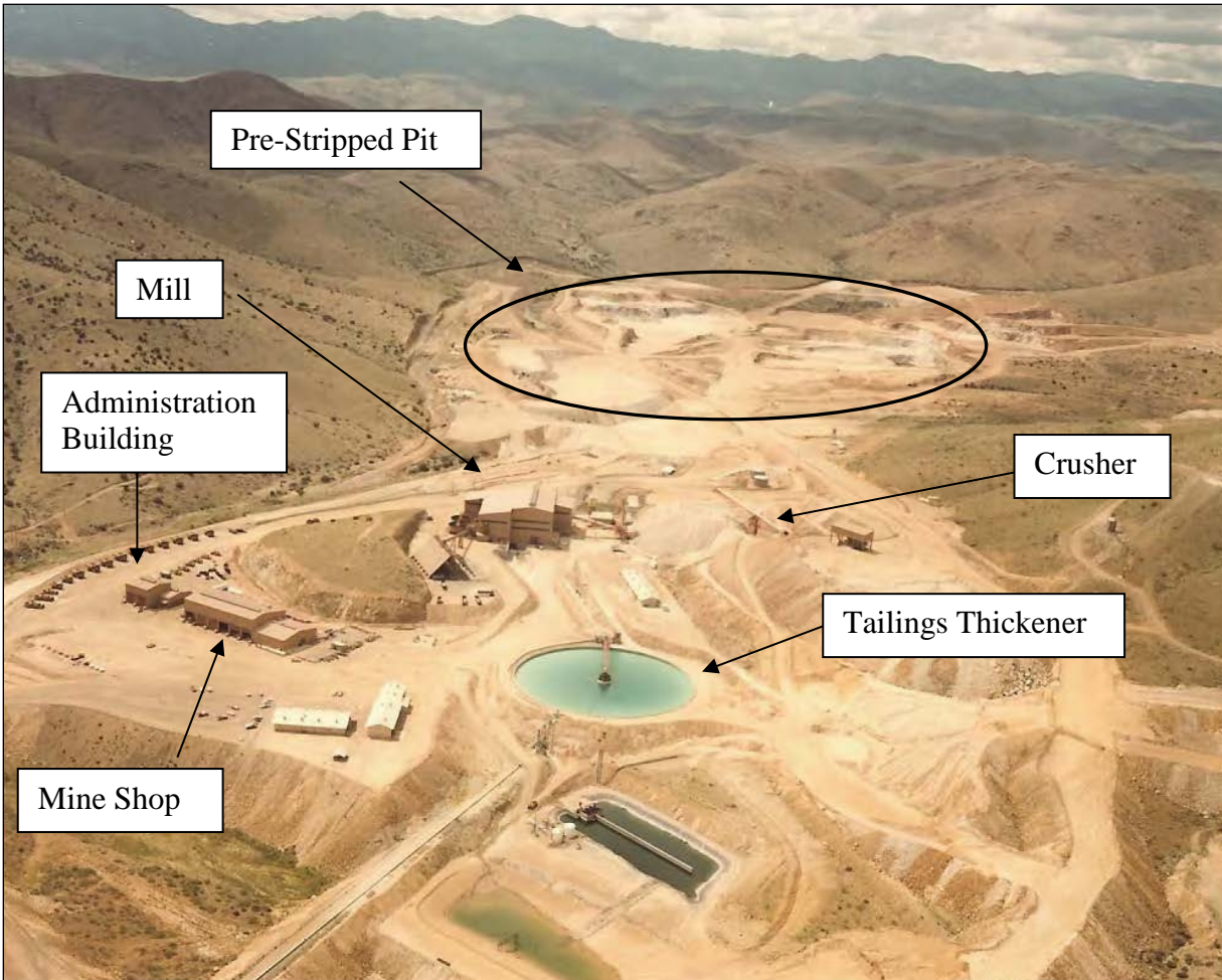
Figure 6-1: Copper Flat Mine in 1982
