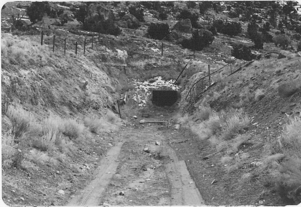
Photo (e) Looking eastward in trench leading to sec. 34 adit sealed with plate metal door.
