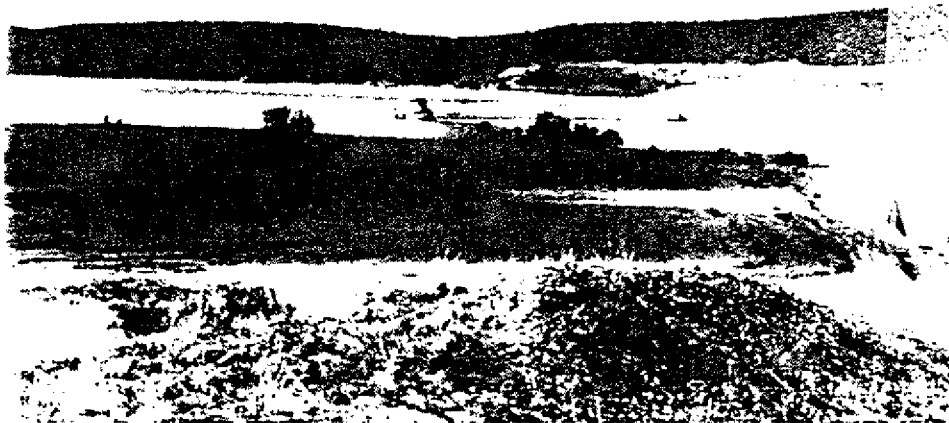
Photo 4. Capping of Tailings Ponds with Soil. (Notice airborne soil; tailings not airborne.) View to southwest. Photo by Stuart Kent.
