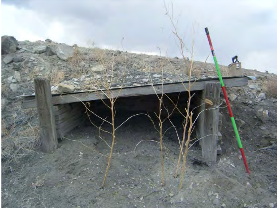
Photo 13-Looking west at the structure (StructPly-1) on the northeast side of PilePly-4.
