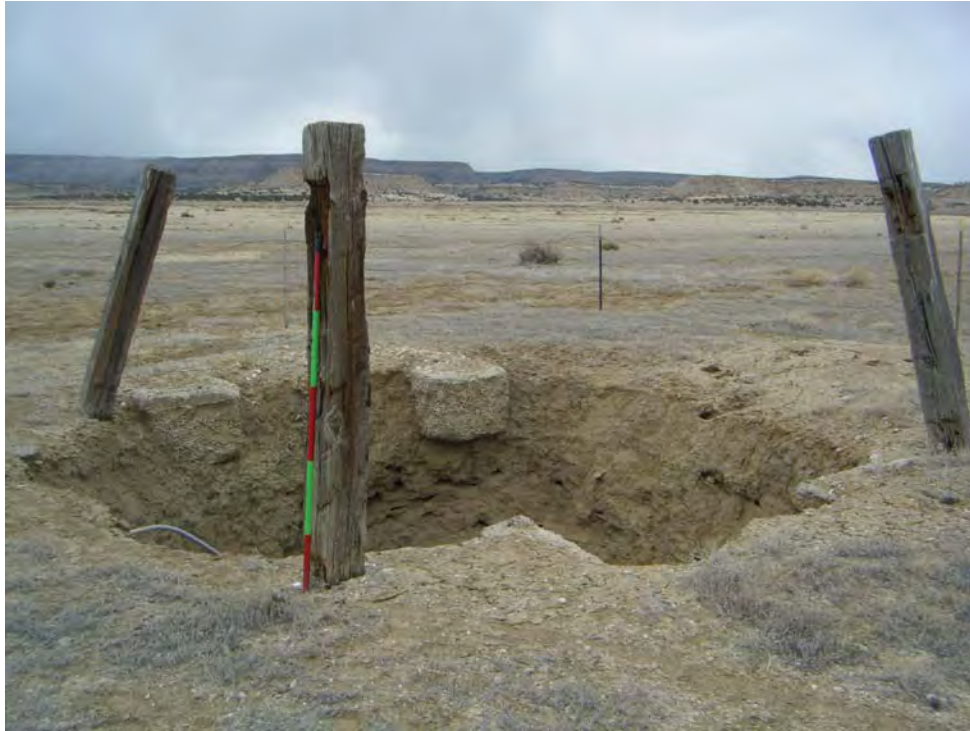
Photo 17-Looking north at a caved mine shaft (ShaftPly-1).
