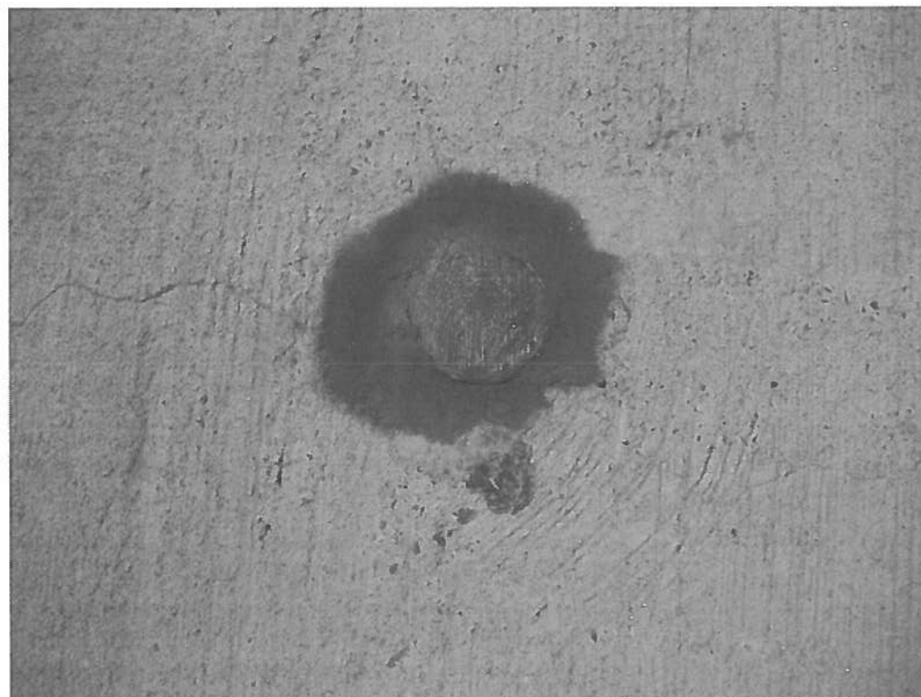
Photograph 4. View of MW-1 approximately 2 hours after placement of cement grout.
