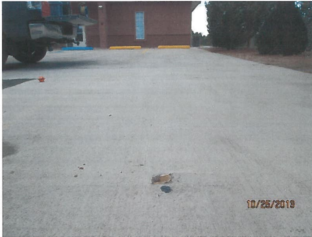
Photograph 1. View of monitor well MW-1 casing in concrete pavement (pre-abandonment).
