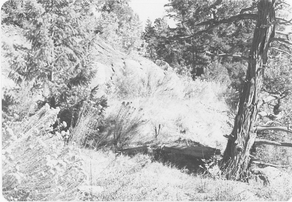
Photo (a) Looking east at the bulldozer cut on the Whiteflow workings.
