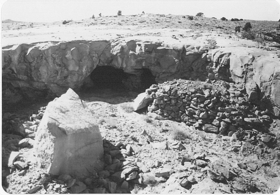
Photo A - Looking SW at twin adit entrance in SW corner of workings. Note stacked waste rock; entrance about 5' high.
