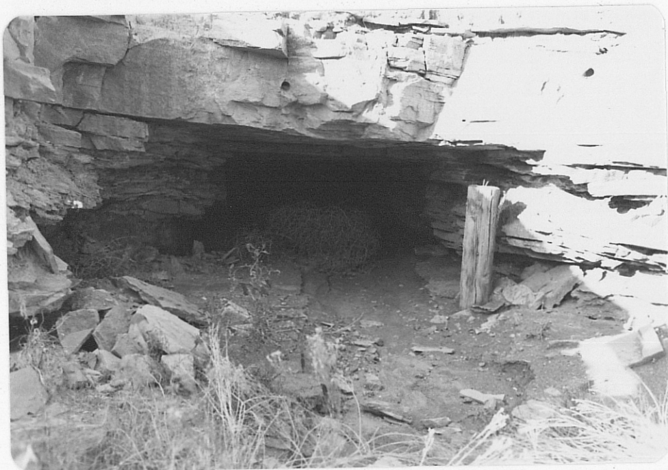
Photo (b) Tent Mine; portal is presently only 3' high by 7' wide.
