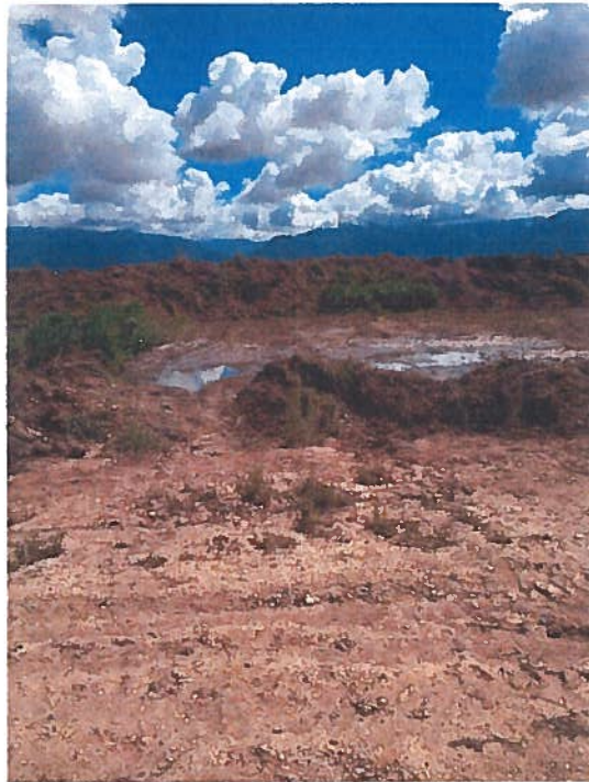
Figure 3: Septic cell with fresh dirt work and some ponding
