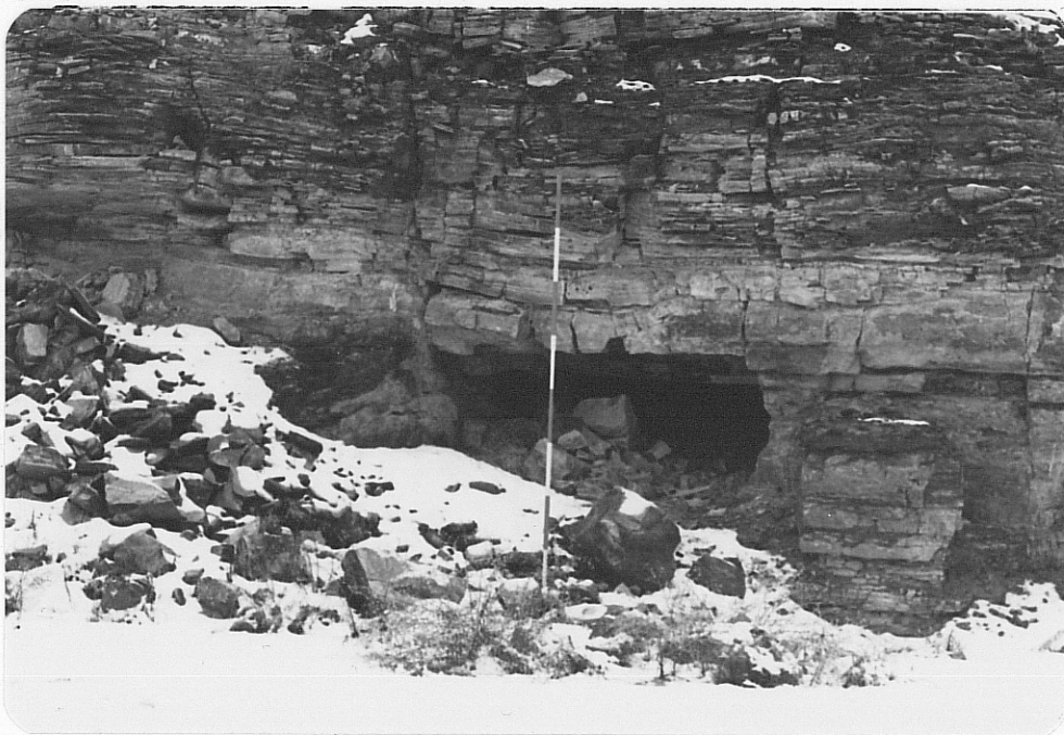
Photo (e) Looking southward; close-up of adit driven in southern face of cut.
