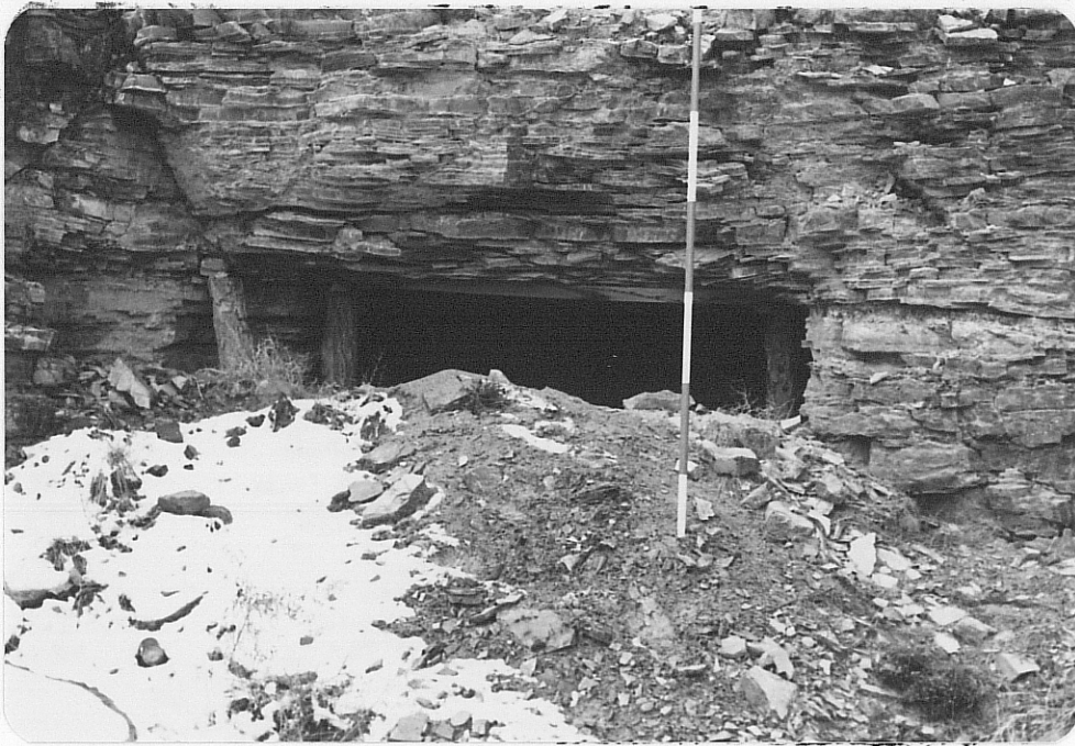
Photo (d) Looking westward; close-up of adit driven in western face at cut.
