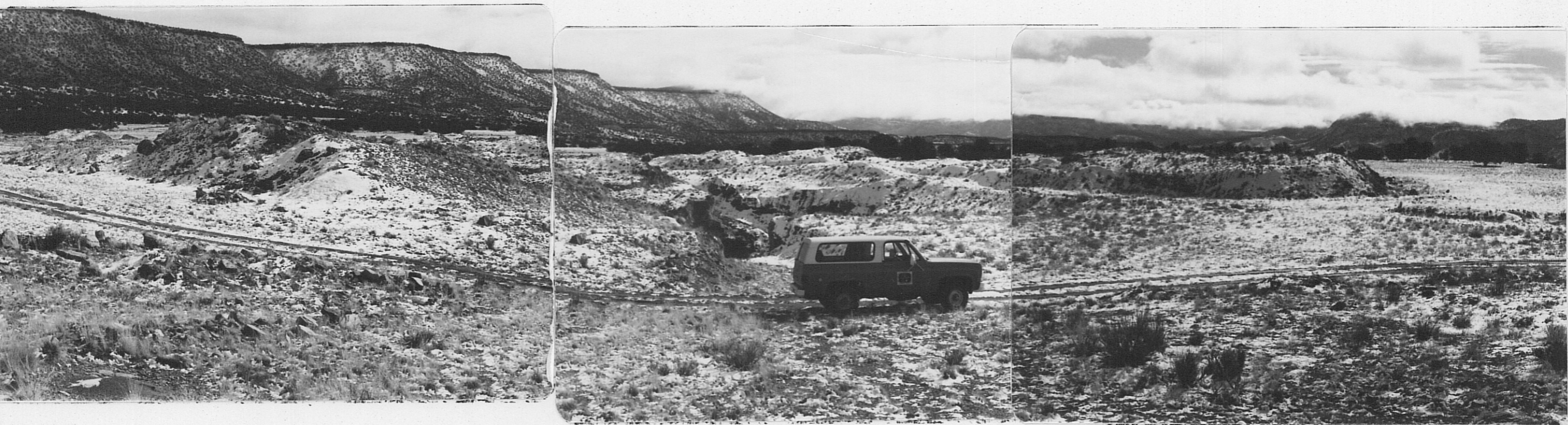
Photo (a) Looking eastward at Zia Mine; open pit at center is 30' deep. La Jara Mesa in background at left. Photo taken after a light snow had fallen.
