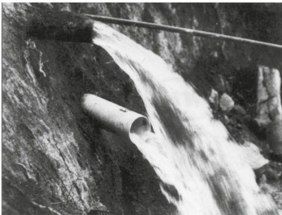
Fig. 17.5 Example of horizontal wells tapping weathered andesite at a height of 2400m above m.s.l. in the Lake Tahoe Basin, California, USA. (After Matthews 1985)
