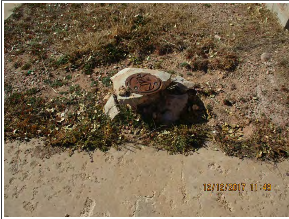
1. Monitor well MW-3 prior to replacement of surface completion.
