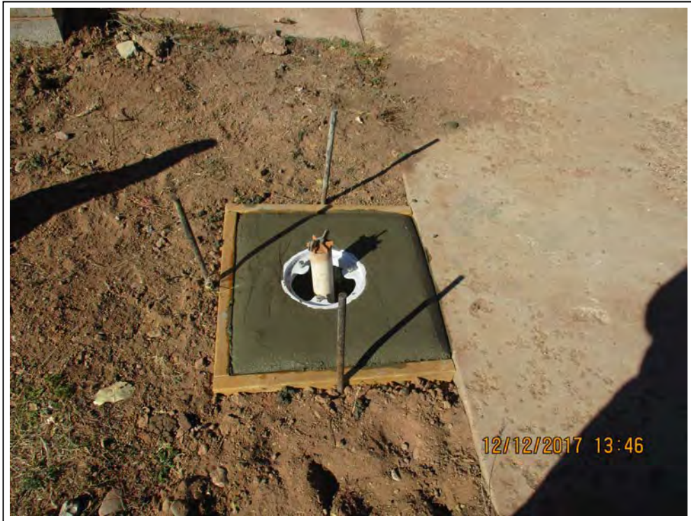
5. MW-3 surface completion prior to cutting off well casing.
