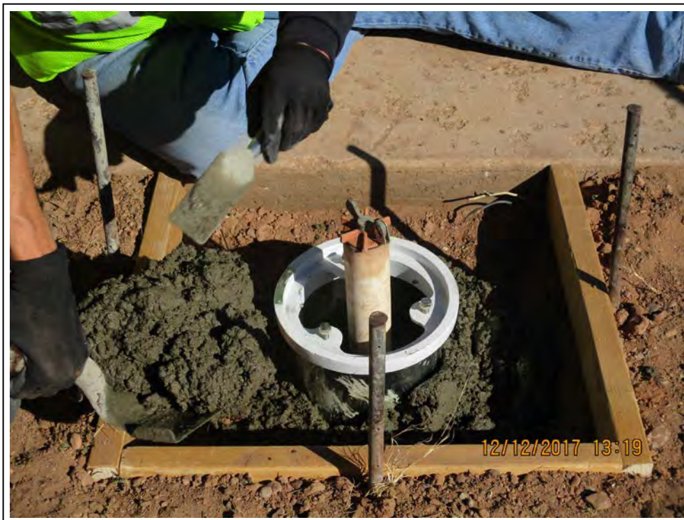
4. Constructing new concrete pad for MW-3.
