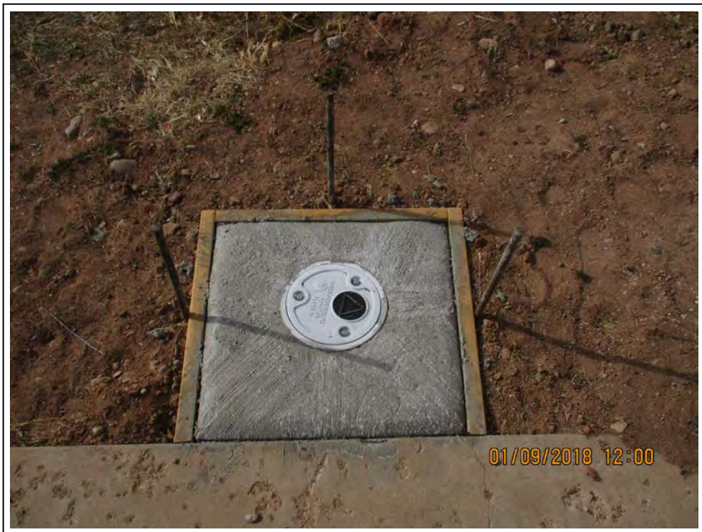
6. Final MW-3 surface completion.
