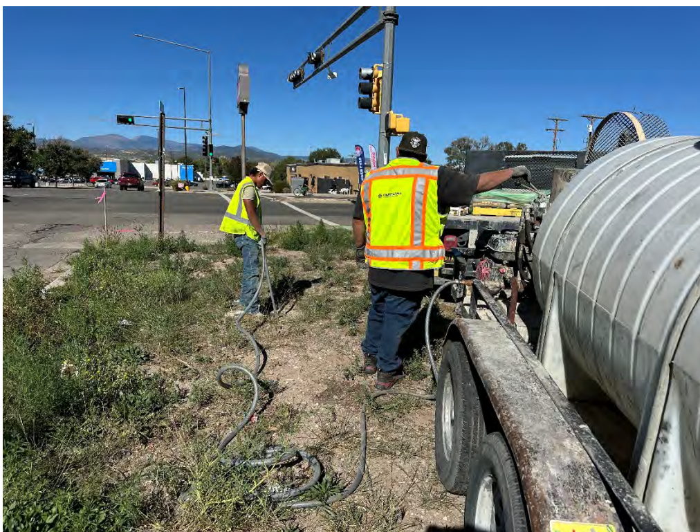
Photo 4. Enviro-Drill placing grout in MW-23, looking west
