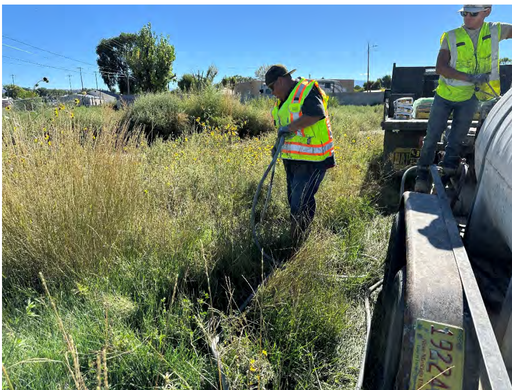
Photo 6. Enviro-Drill placing grout in MW-22, looking west
