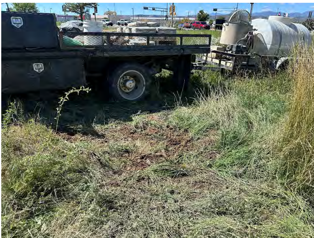
Photo 10. MW-22 location returned to grade, looking southwest
