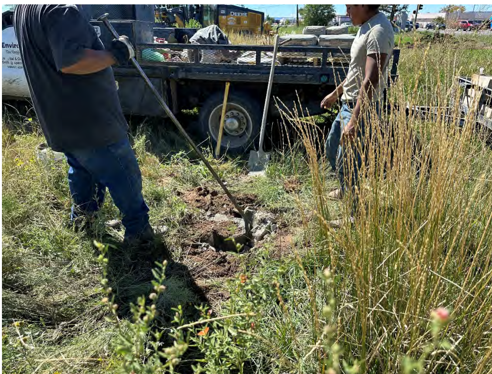
Photo 9. Enviro-Drill removing MW-22 surface completion, looking southwest
