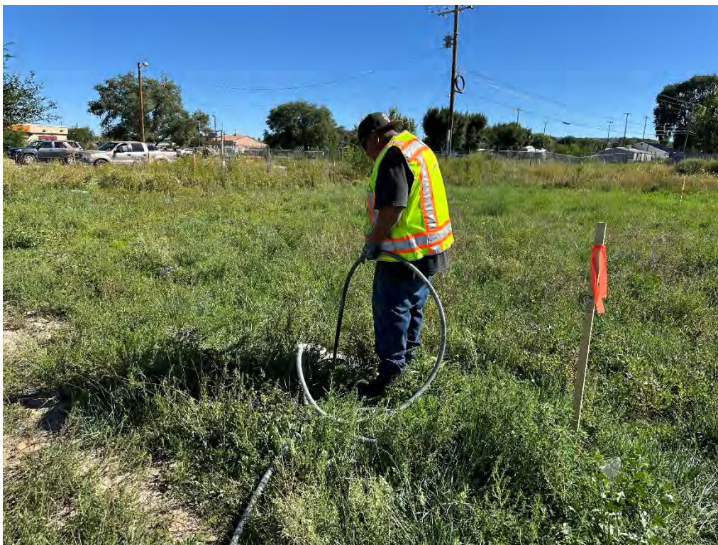
Photo 5. Enviro-Drill placing grout in MW-13, looking northeast
