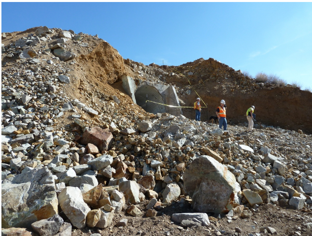
Photo 1 – Entrance to Steel Tunnel
