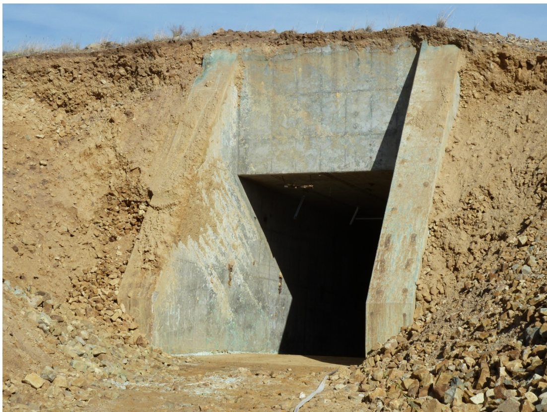
Photo 6 – Stockpile Entrance – Conveyor Gallery
