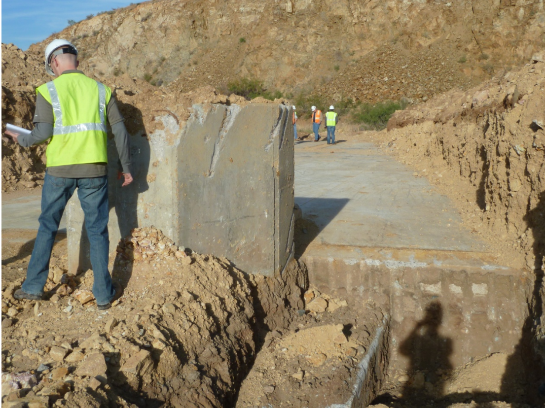
Photo 15 – Truck Shop Floor Slab
