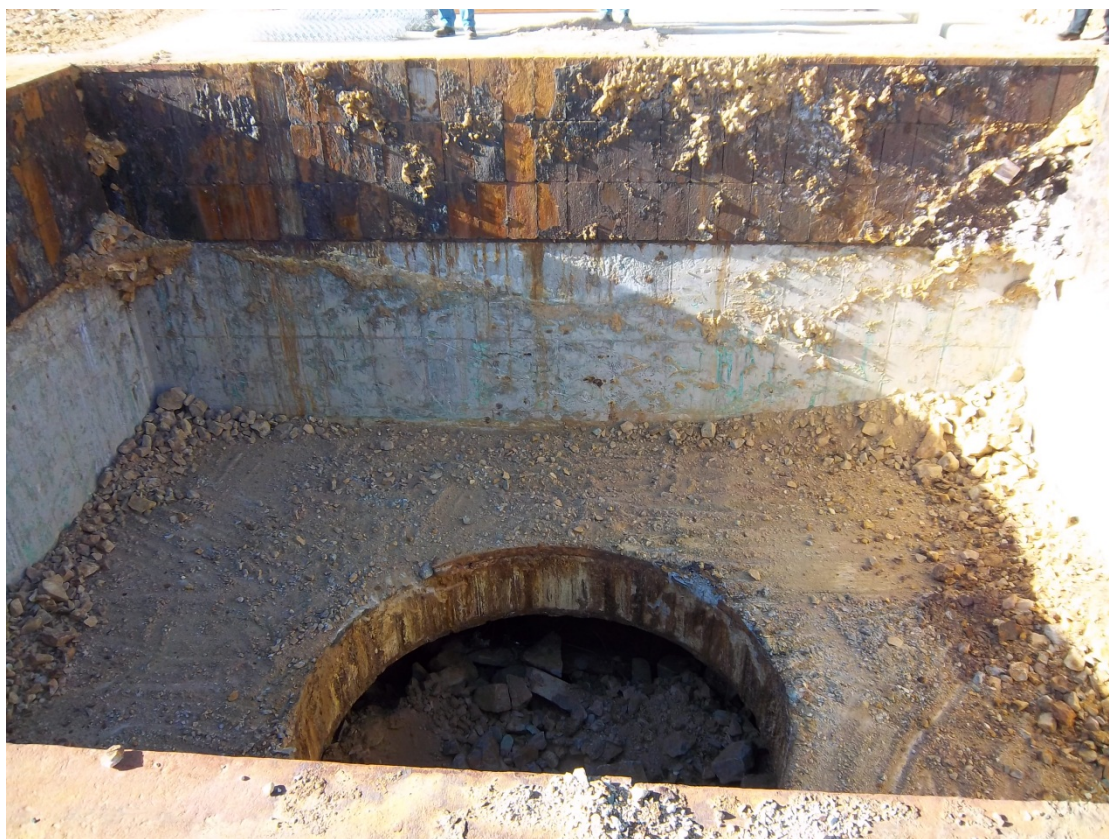
Photo 1 – Primary Crusher - Excavation Progress on Crushing Side
