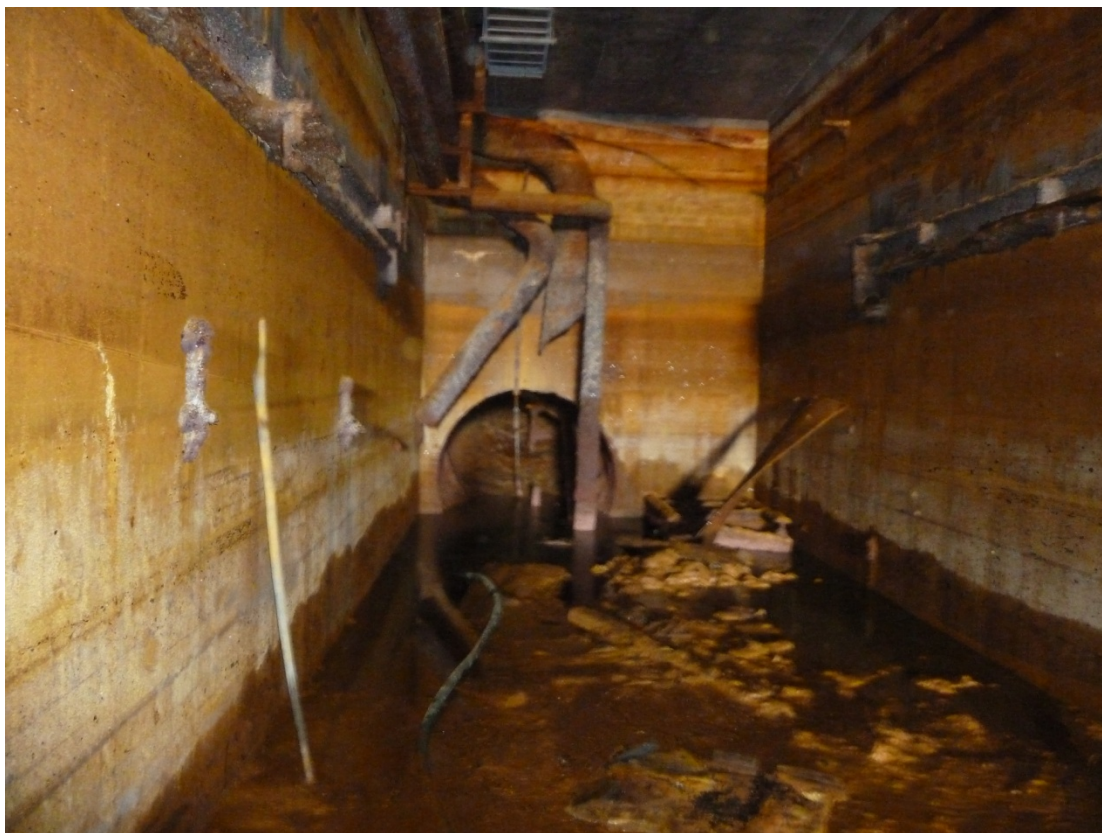
Photo 9 – Escape Tunnel from Vault
