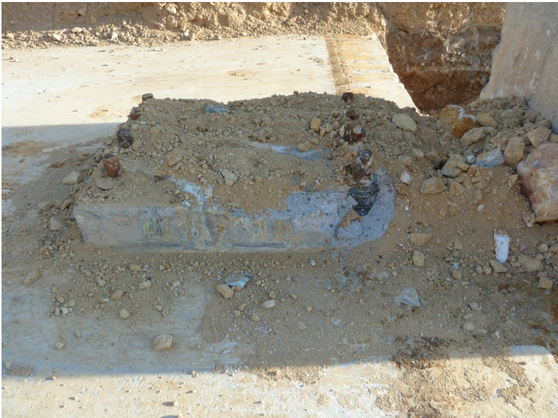
Photo 16 – Truck Shop, Typical Column Foundation
