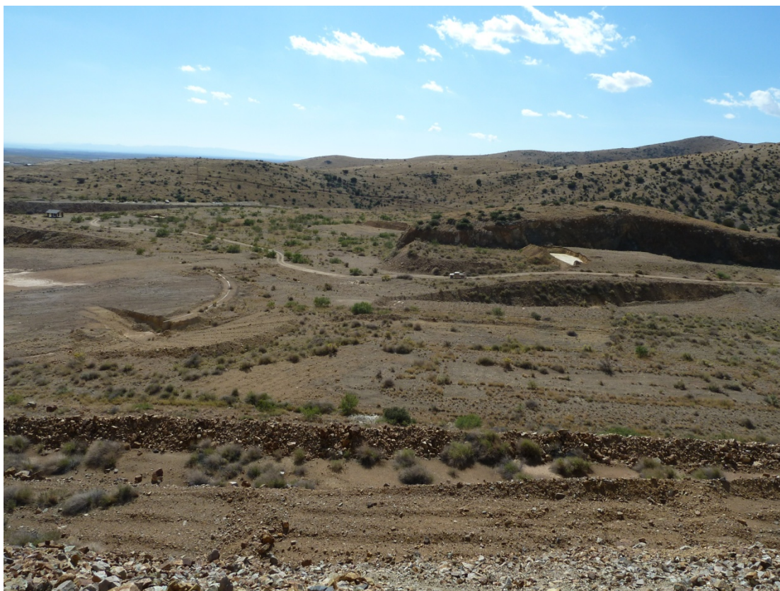
Photo 18 – Concentrator Stockpile Slab from Primary Crusher
