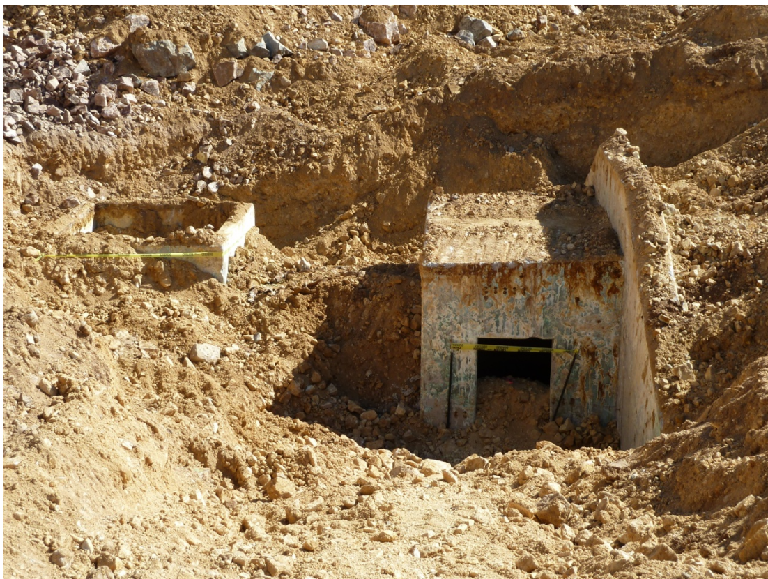
Photo 10 – Reclaim Tunnel Escape Manway and Valve Box
