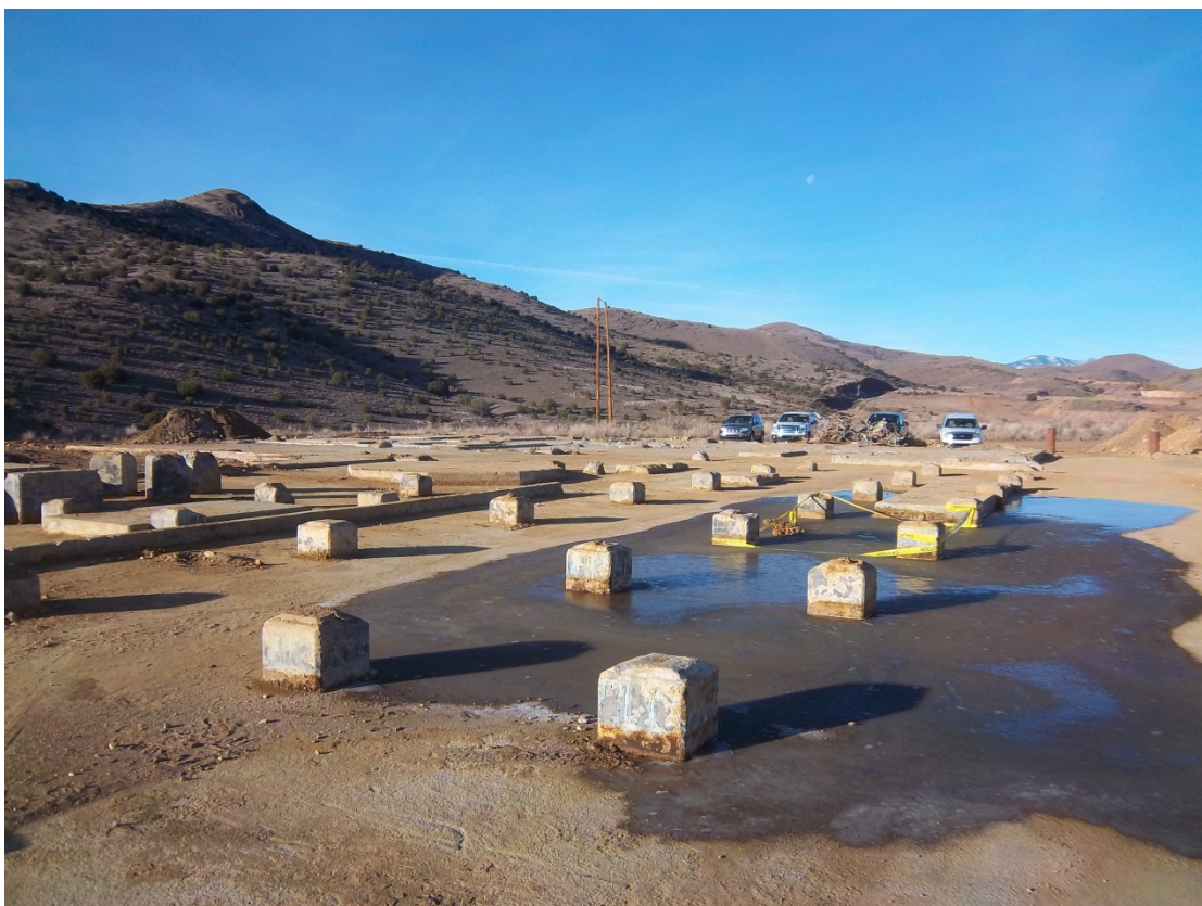
Photo 8 – Flotation Area – Existing Interior Concrete Piers
