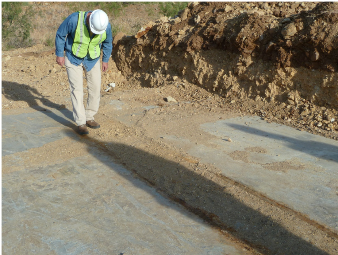
Photo 17 – Truck Shop – Floor Trench in Electrical Room
