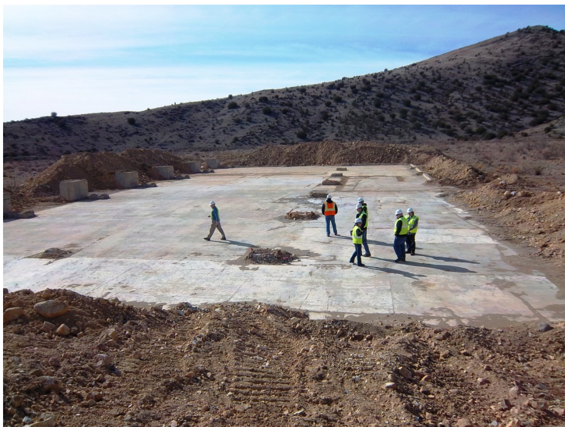
Photo 12 – Truck Shop – Excavation Progress
