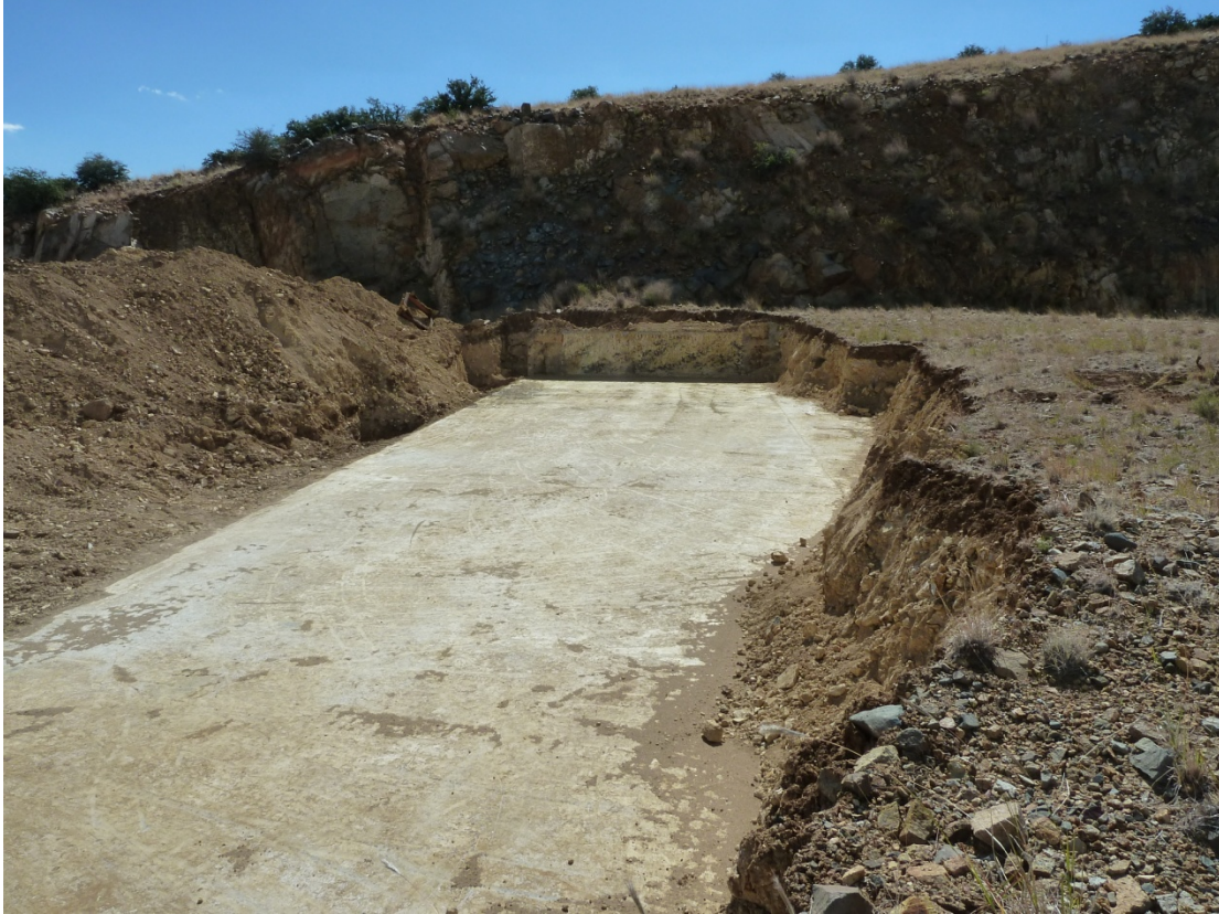
Photo 19 – Concentrator Stockpile With Push Wall at Rear
