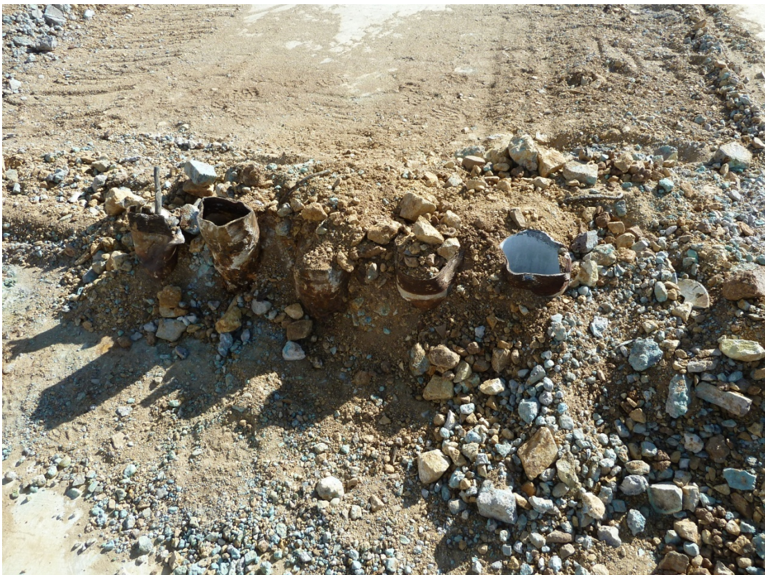
Photo 20 – Underground Utility Floor Penetration
