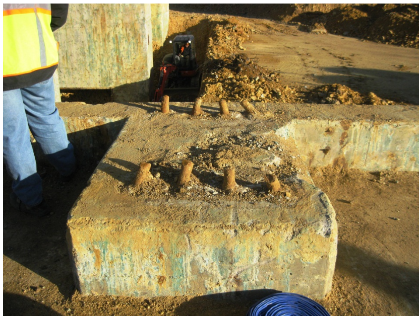
Photo 11 – Concentrator – Typical Building Pier
