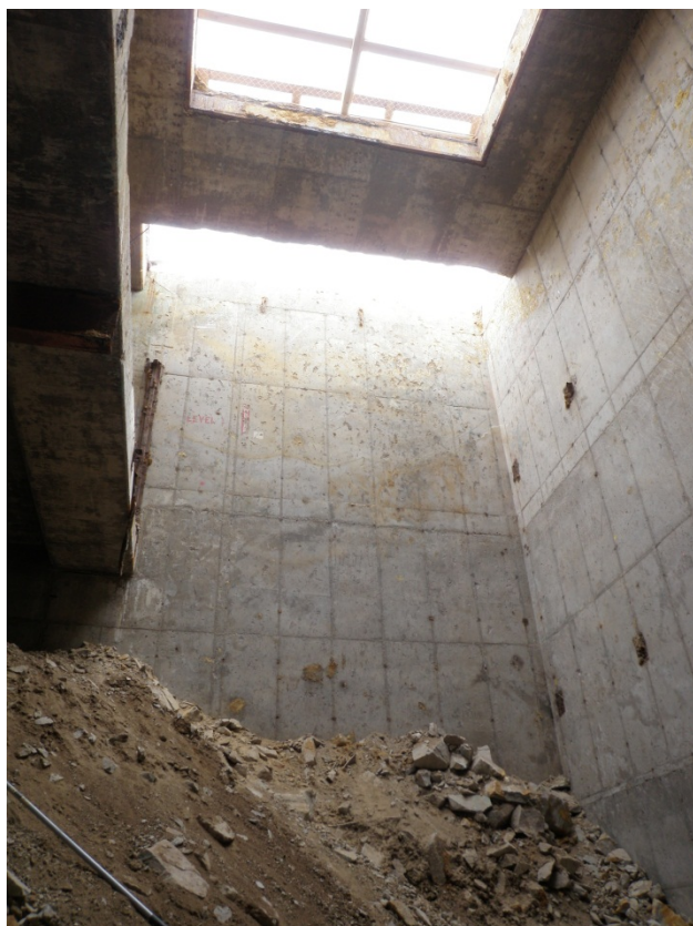
Photo 2 – Primary Crusher – Excavation Progress on Maintenance Side
