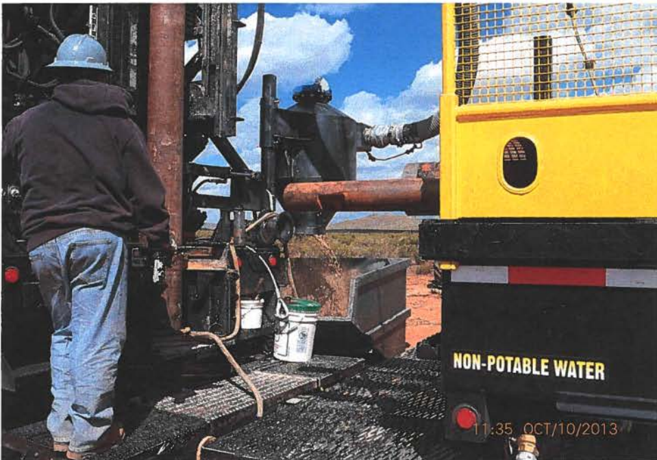
Hing 1st Water
