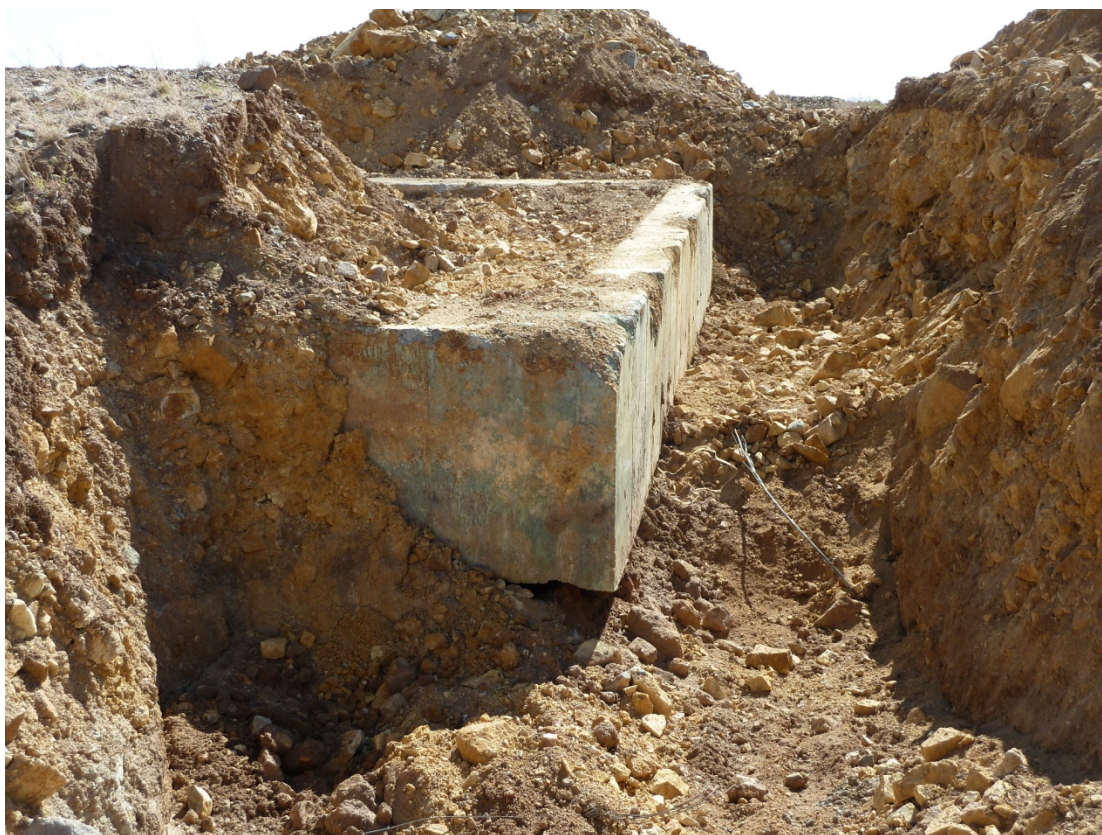
Photo 5 – Primary Crusher – Maintenance Area
