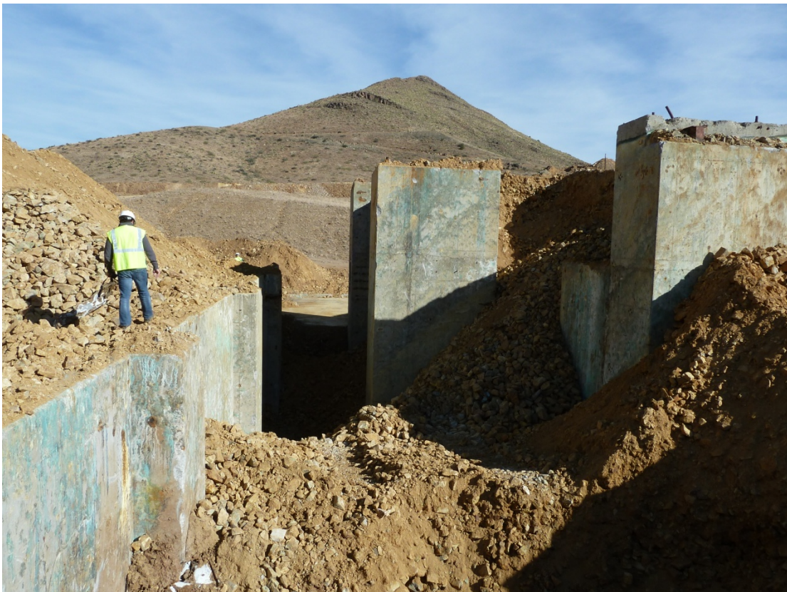
Photo 12 – Concentrator SAG Mill Footings
