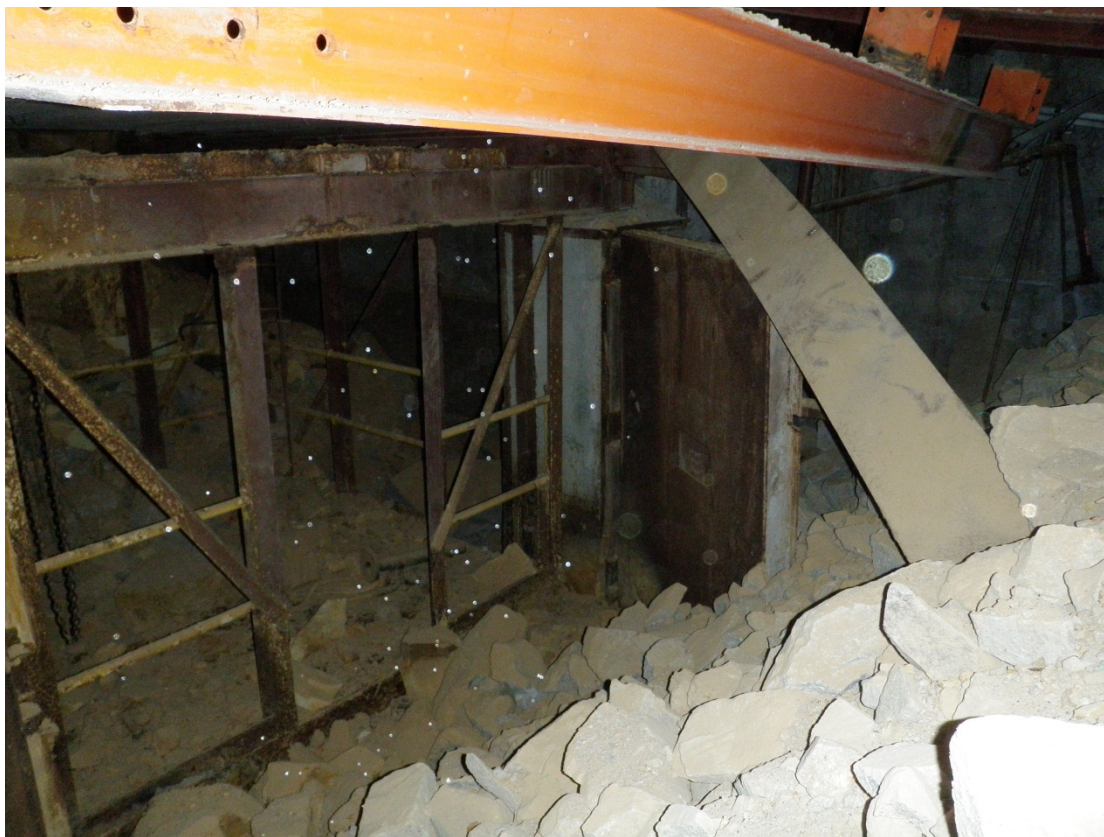
Photo 5 – Primary Crusher – Remains of Structural Steel
