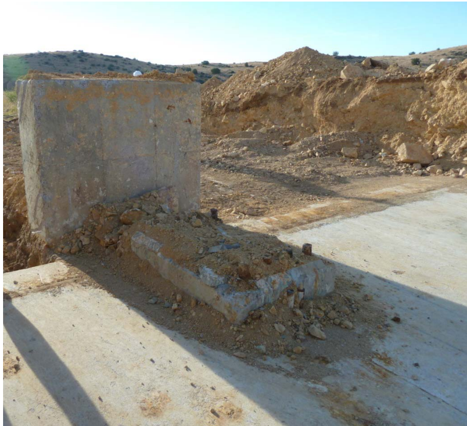
Photo 14 – Typical Column Base at E3
