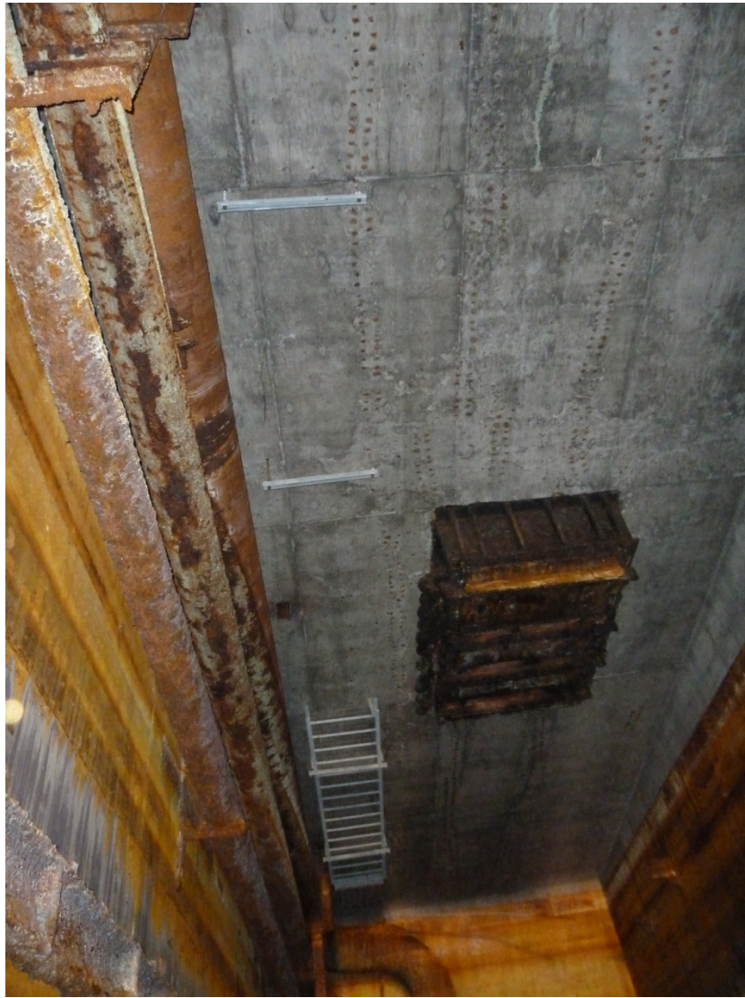
Photo 8 – Draw Hole in Vault Area
