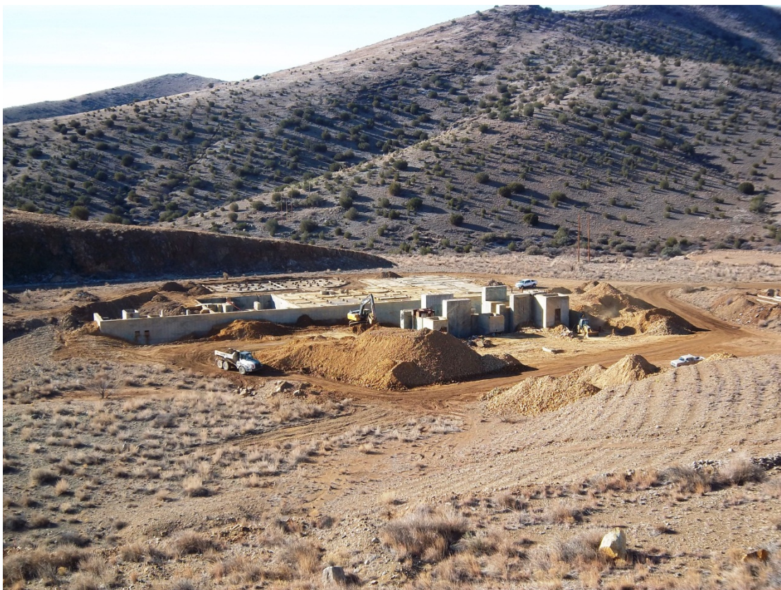
Photo 7 – Concentrator – Excavation Progress
