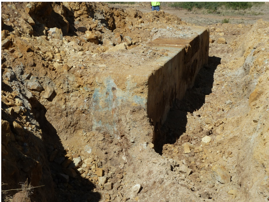
Photo 4 – Primary Crusher Dump Pocket
