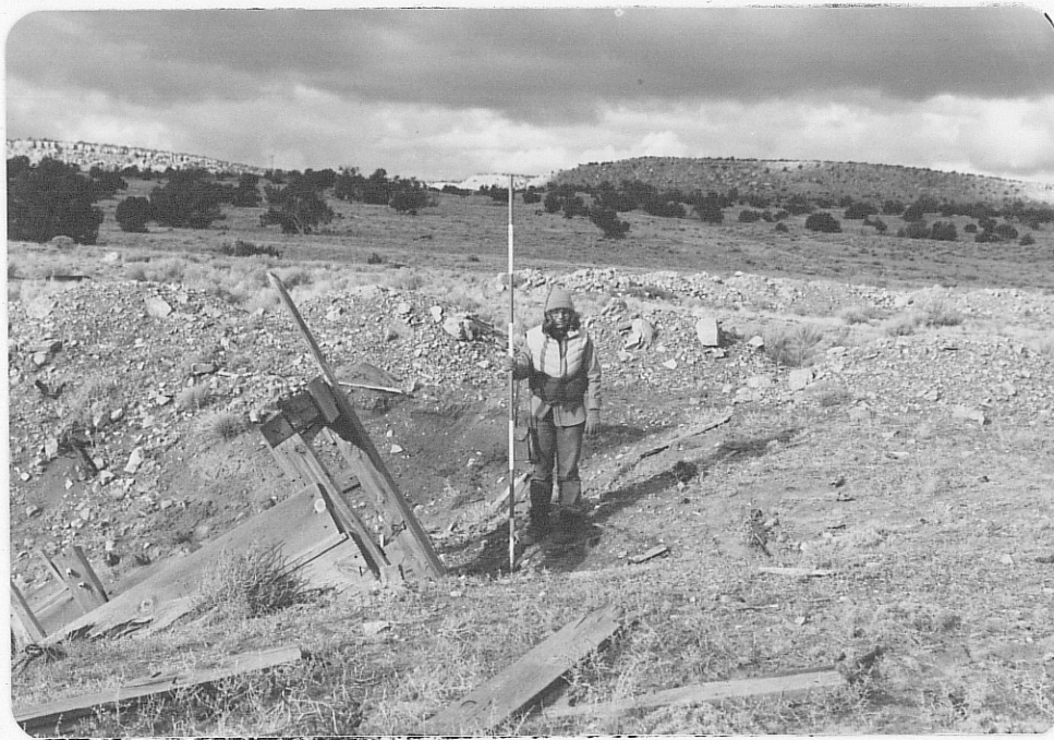
Photo (a) Looking north at entrance to incline; shaft slopes off to left at 30^{\circ} .
