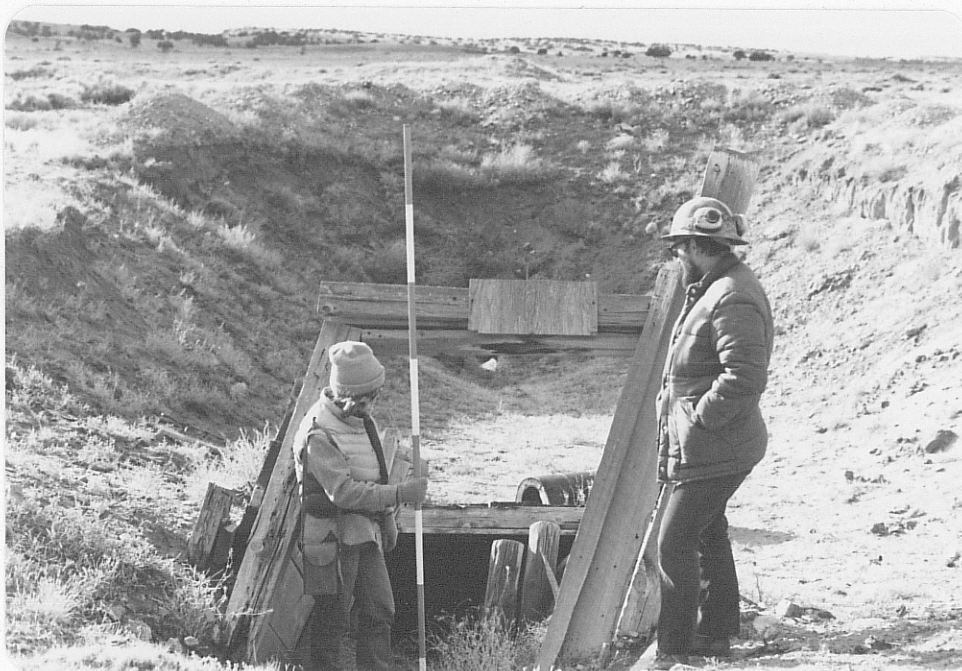
Photo (b) Looking west into entrance showing 2\frac{1}{2}' high opening that remains; natural processes are filling in portal area. Note scattered waste piles in background behind box cut.
