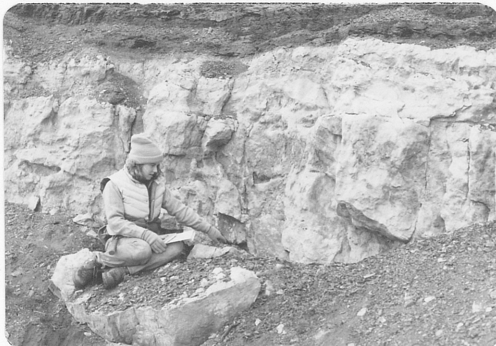
Photo (b) Caving at portal of adit near center of cut shown in photo (a); person is pointing to remaining small opening.
