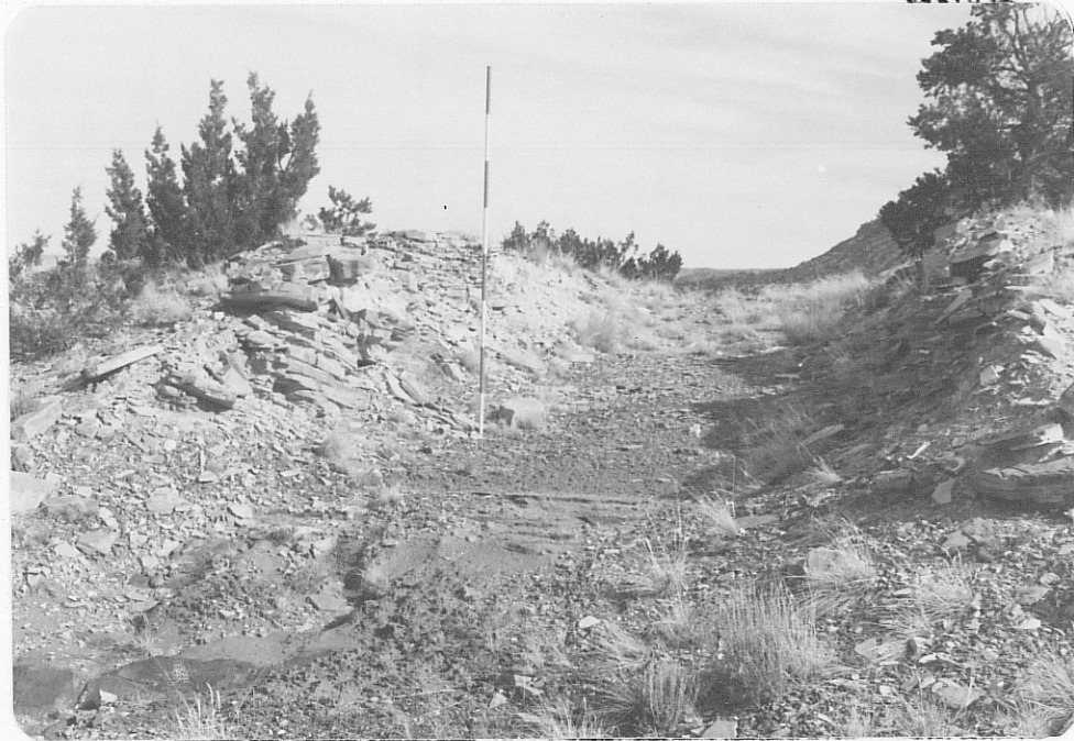
Photo (a) Looking northeastward into 40' long prospecting trench, 3' deep.
