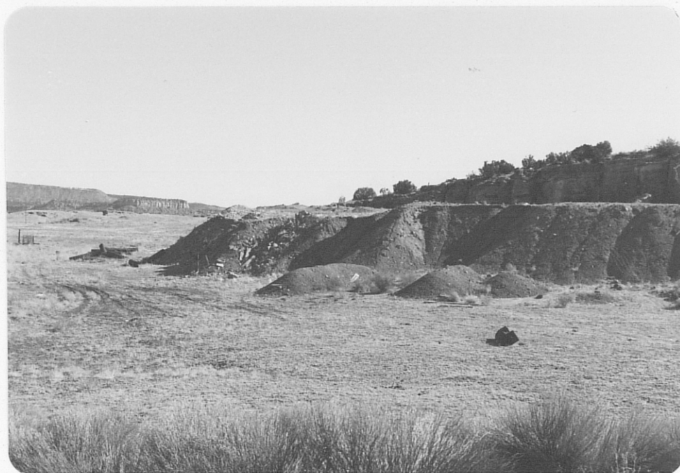
Photo (f) Looking east at southern edge of tailings dump. San Mateo Creek lies 400' to south; portal is at base of sandstone cliff behind dump at right.
