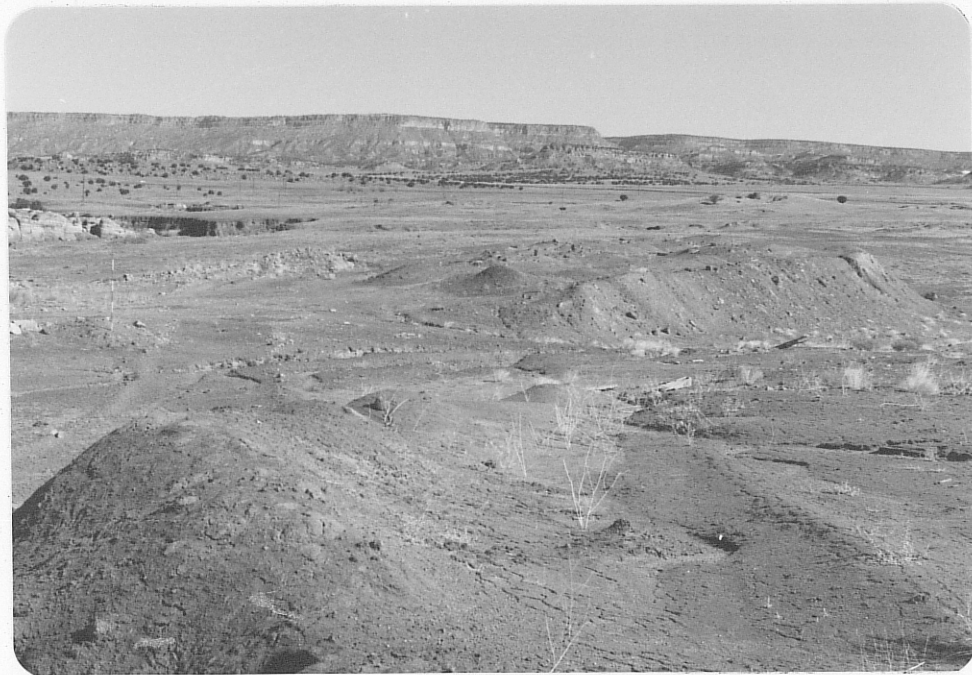
Photo (d) View eastward on upper surface of tailings dump showing ramp ascending from mine level at center right; note range pole at far left for scale.
