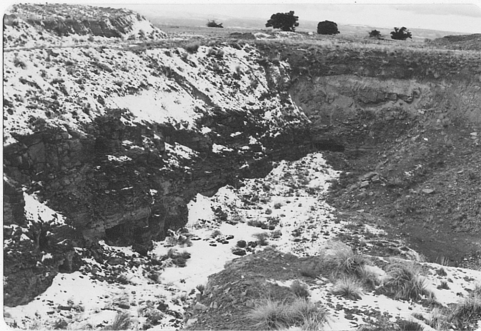
Photo (c) Looking westward from nearly same point as in photo (b), but both adits at bottom of cut are shown here.
