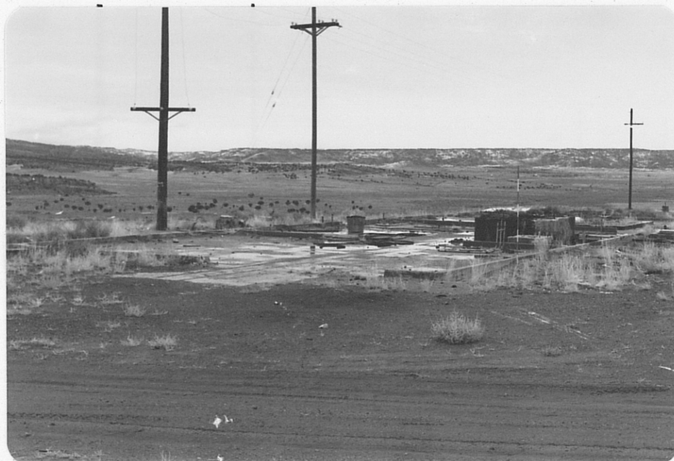
Photo (f) Looking northeastward at concrete slab and hoist and drum foundation. Slab measures 38' x 115'; note range pole for scale.
