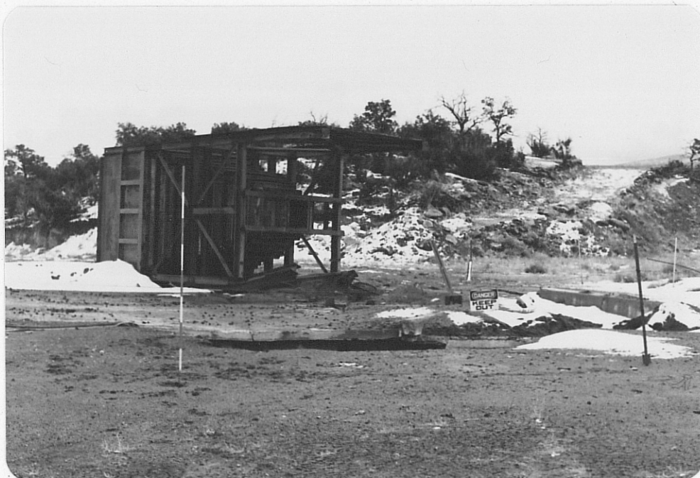
Photo (b) Looking northeast at shaft site showing caving which has begun around perimeter of concrete slab, and toppled ore bin; note range pole for scale.
