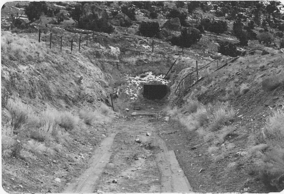
Photo (e) Looking eastward in trench leading to sec. 34 adit sealed with plate metal door.
