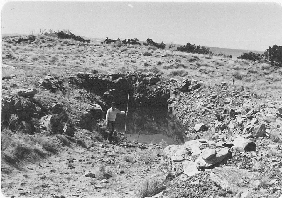
Photo (c) Looking west into workings near Red Bluff #4 and #5 boundary; this pit is probably on the Red Bluff #4 side. Pond is 10' wide, 25' long, and 2\frac{1}{2} ' deep at maximum.
