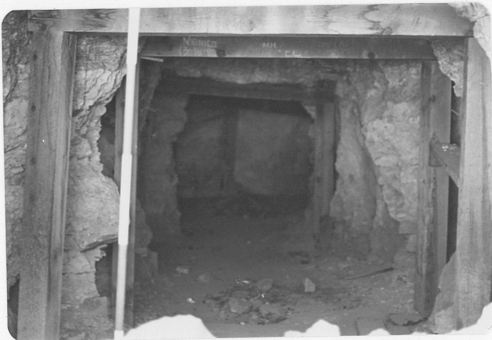
Photo (c) View inside western adit; note timbering, grafitti, campfires, and split into left and right forks at rear.
