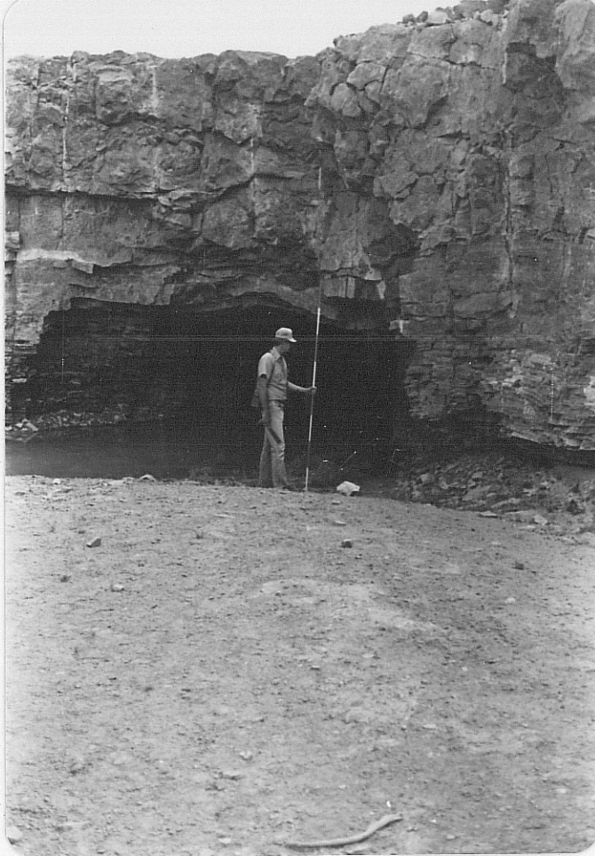
Photo (b) Looking southeastward from floor of open pit into 7' high, 10'-12', adit shown at right in photo (a).
