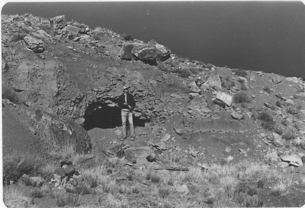
Photo (a) Looking eastward at 6' x 8' portal of adit at Chavez Mine. Maximum scintillometer readings were obtained at left side of portal where person is standing.
