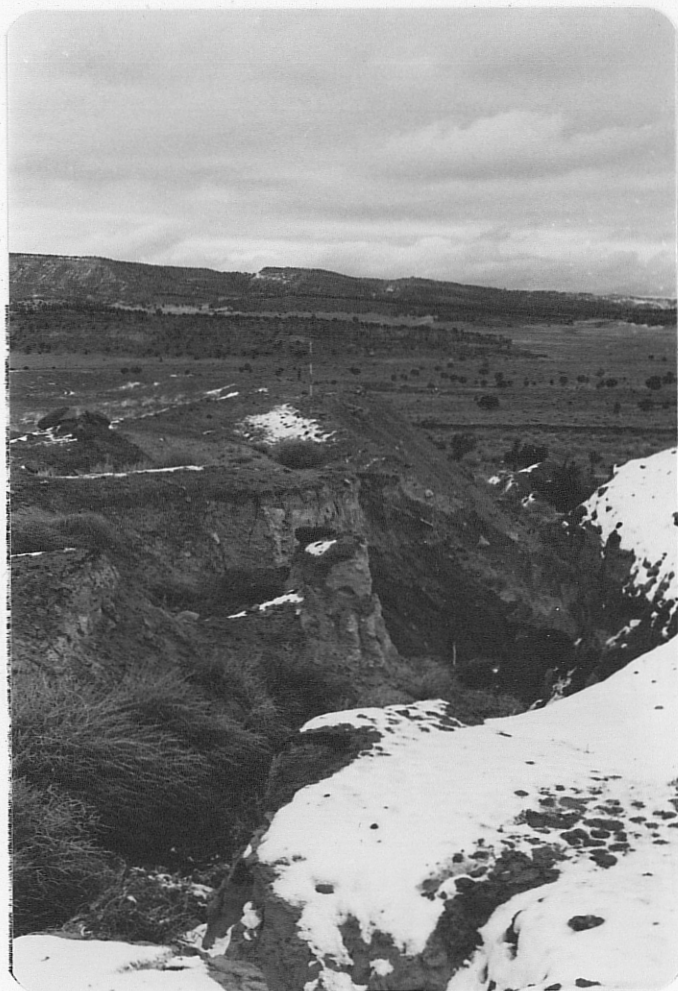
Photo (i) View northward at east edge of dump showing gullying; note range pole for scale and tributary in background visible through the gully notch.
