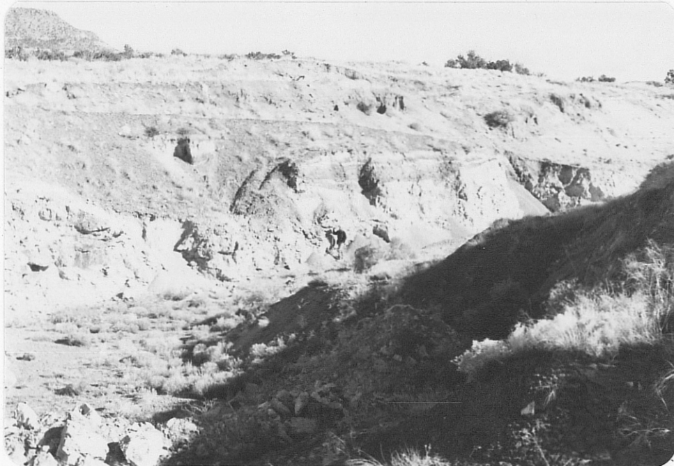
Photo (12) Southern extension of cut shown in (11) above. Road surface descends to right on bench in background. Note person in center photo for scale.
