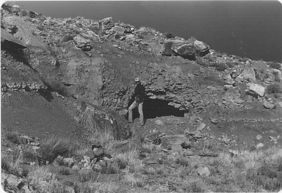
Photo (a) Looking eastward at 6' x 8' portal of adit at Chavez Mine. Maximum scintillometer readings were obtained at left side of portal where person is standing.
