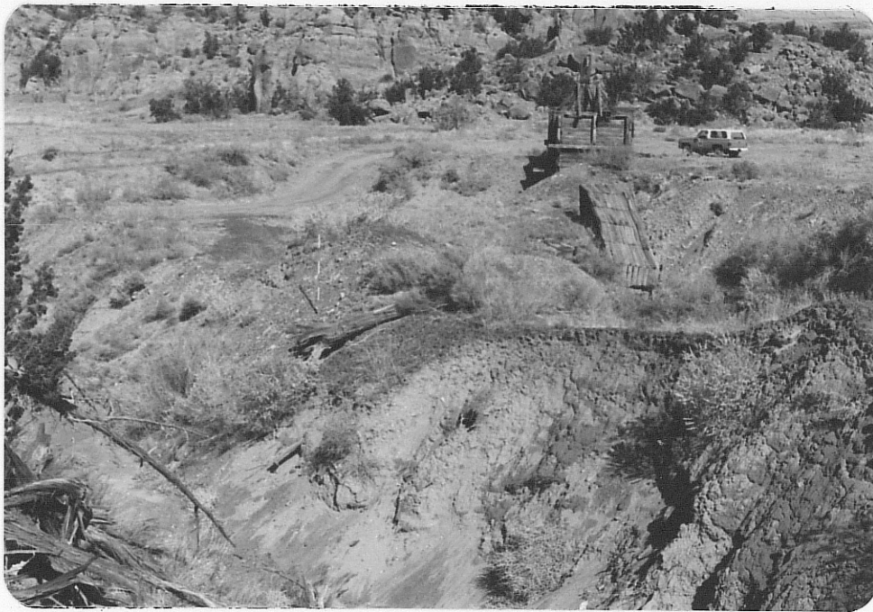
Photo (b) View northward of timbered incline and the headframe and loadout, from drainage line; range pole is on narrow divide between drainage line and caved area over the incline.
