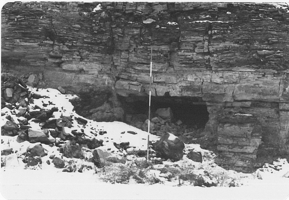
Photo (e) Looking southward; close-up of adit driven in southern face of cut.
