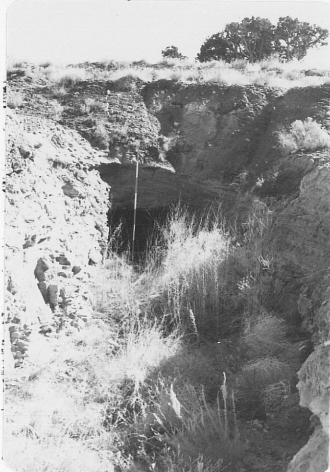
Photo (f) Looking southeastward into small adit 4' high, 6' wide, 20' long near the southwest end of the Red Bluff #2 Claim.
