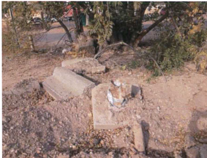
Photograph No. 2 Well vault for MW-1R located in a pile of construction debris approximately 10 feet from location of Well casing for MW-1R
