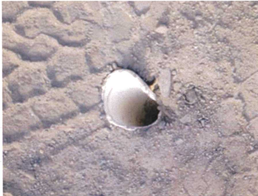
Photograph No. 12 PVC well casing for RNMW-2 located; casing bent approximately 1 foot below ground surface.
