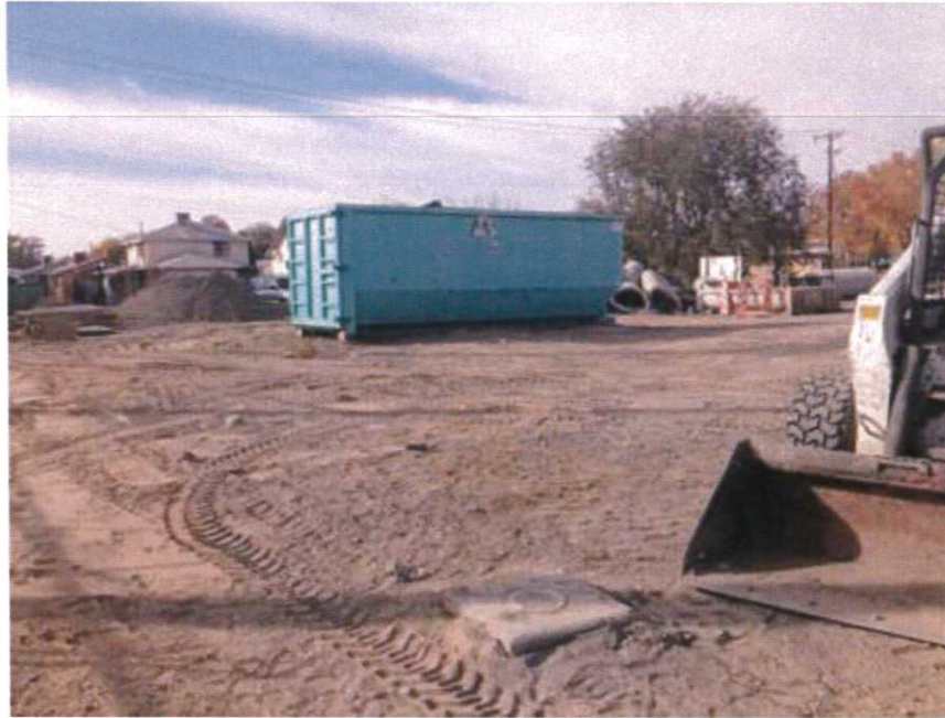
Photograph No. 19 Former location of MW-6R, looking west-northwest. Well MW-4R in foreground.
