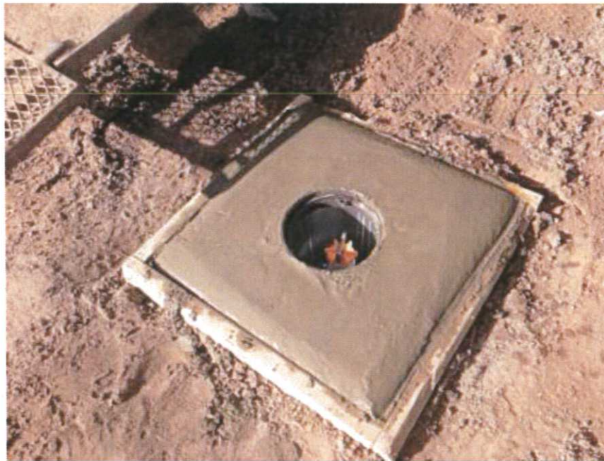
Photograph No. 21 Well vault and concrete pad for newly installed MW-6RR.
