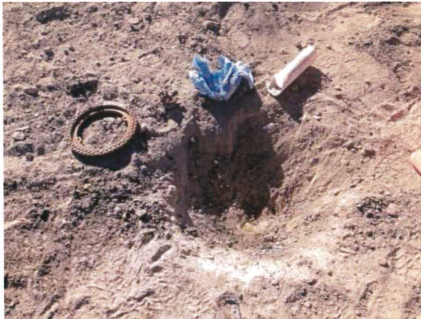
Photograph No. 14 Left to right: Steel ring used to mark location of well for metal detector use, plug made from rag attached to wire, remains of upper portion of casing from RNMW-2
