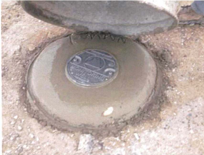
Photograph No. 9 New well vault and concrete pad for NMW-1.
