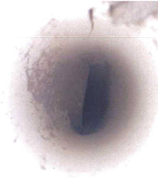
Photograph No. 13 Close-up view of bent casing in RNMW-2.
