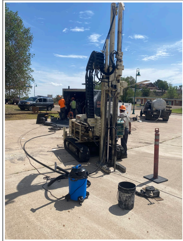
4. Geoprobe and trailer (view to southeast)
