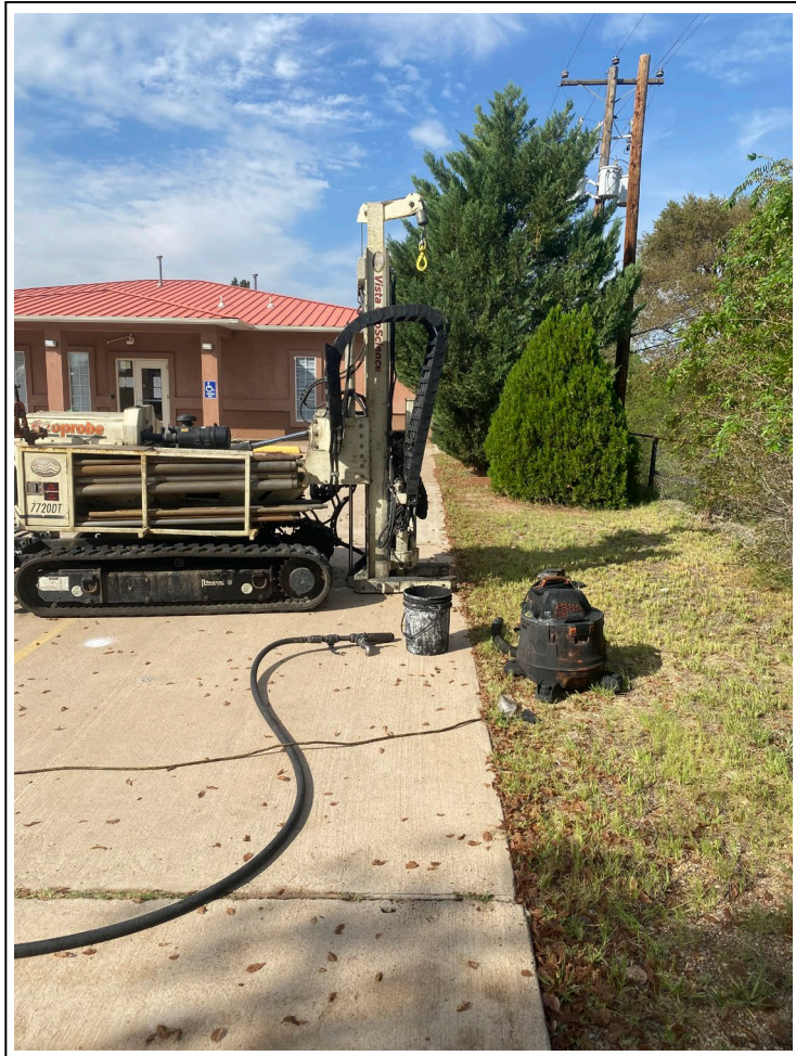
1. Vista set up to begin injection at IP-2
