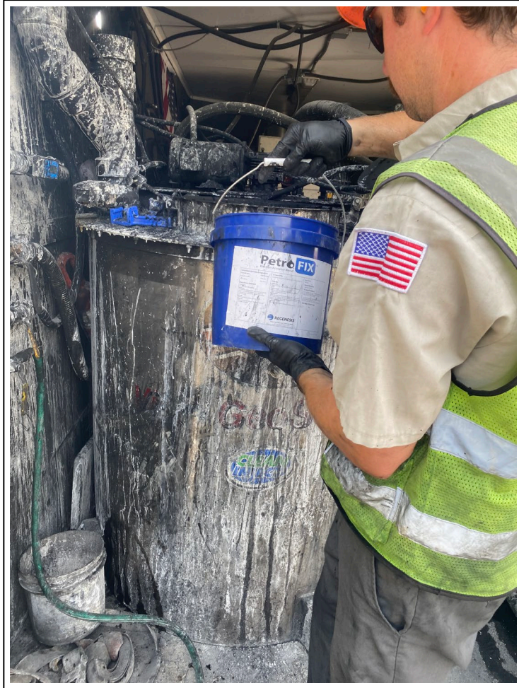
3. Vista personnel preparing PetroFix for injection
