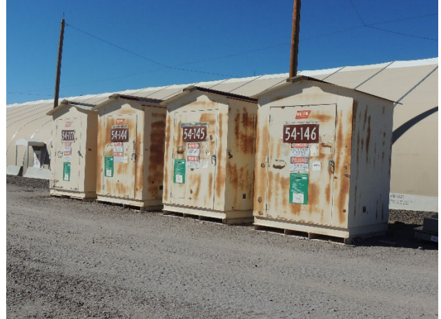
TA-54-144, TA-54-145, TA-54-146, and TA-54-177, Storage Sheds Area G, Consolidated Pad No. 5 (Formerly Pad Nos. 5, 7, and 8) Process Code S01, Container Storage
