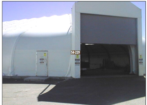
TA-54-229, Area G, Pad No. 9 Storage Dome Process Code S01, Container Storage Process Code T04, Other Treatment
