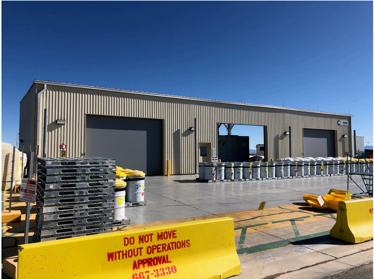
TA-55-0355 Pad Process Code S01, Outdoor Container Storage
