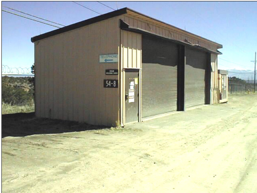
TA-54-8, Area G, Storage Shed Process Code S01, Container Storage Unit
