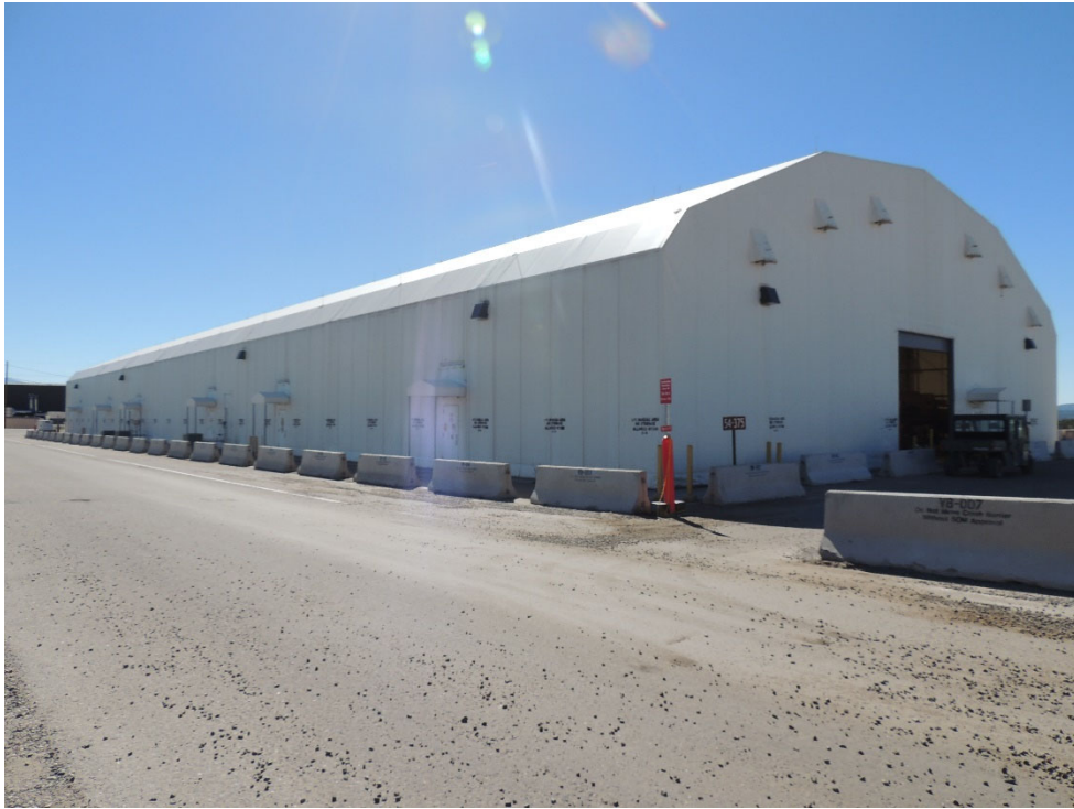
TA-54-375 Storage Dome, Area G, Pad No. 11 Process Code S01, Container Storage Process Code T04, Other Treatment
