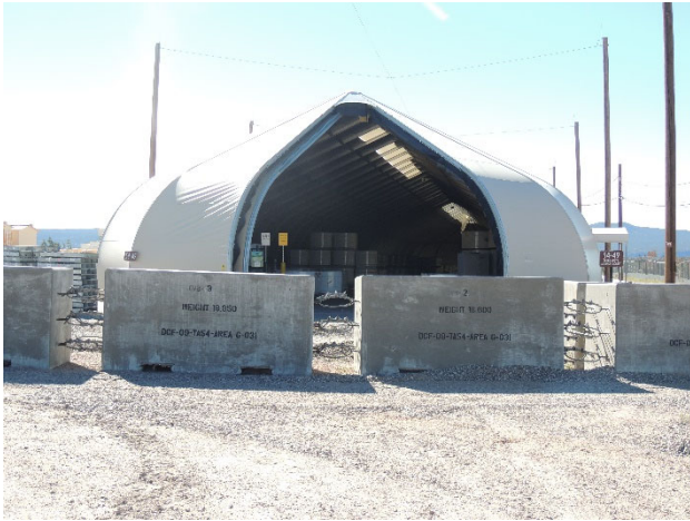
TA-54-49, Storage Dome Area G, Consolidated Pad No. 5 (Formerly Pad Nos. 5, 7, and 8) Process Code S01, Container Storage Process Code T04, Other Treatment
