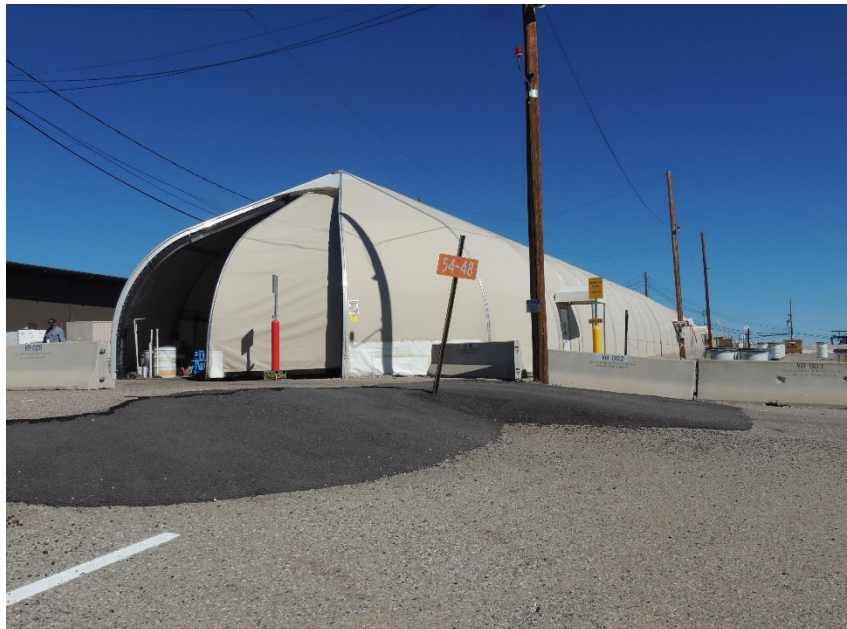
TA-54-48, Area G, Pad No. 3 Storage Dome Process Code S01, Container Storage Process Code T04, Other Treatment
