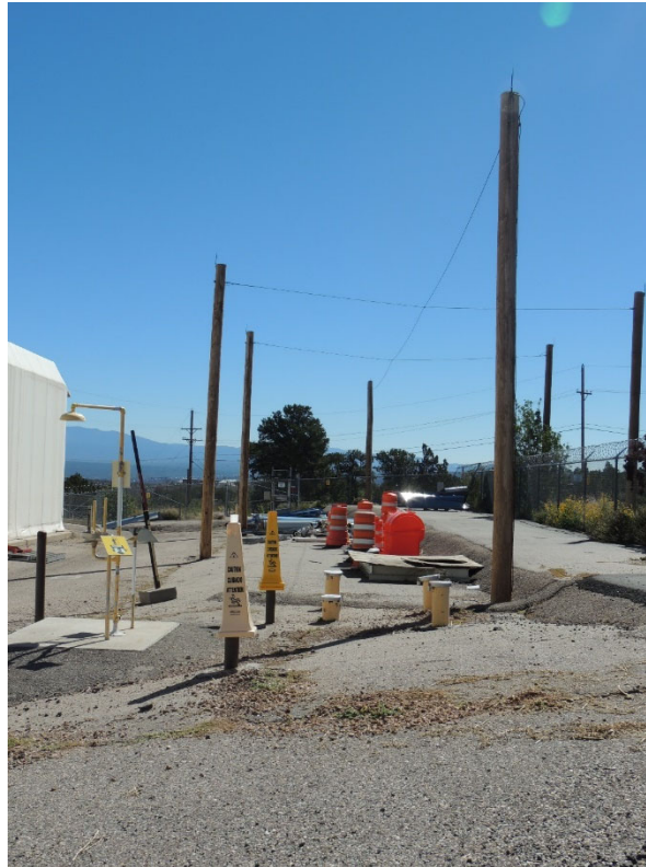
TA-54, Area L, Process Code D80, Disposal Shafts 13-17 and 19-28 (To be closed)
