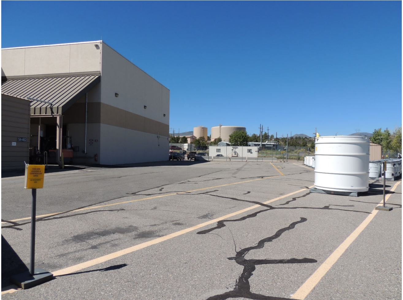
TA-54-38 West Outdoor Pad, Process Code S01, Container Storage Unit Process Code T04, Other Treatment
