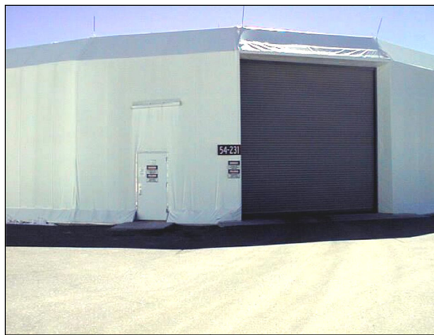
TA-54-231, Area G, Pad No. 9 Storage Dome Process Code S01, Container Storage Process Code T04, Other Treatment
