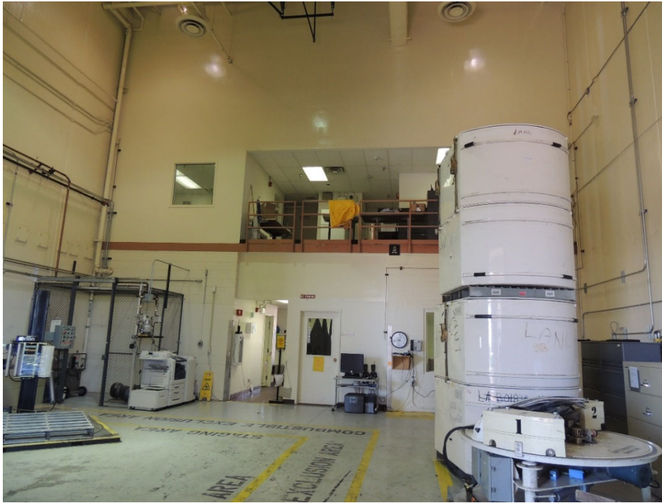
TA-54-38 West Indoor, Low Bay, Process Code S01, Container Storage Unit
