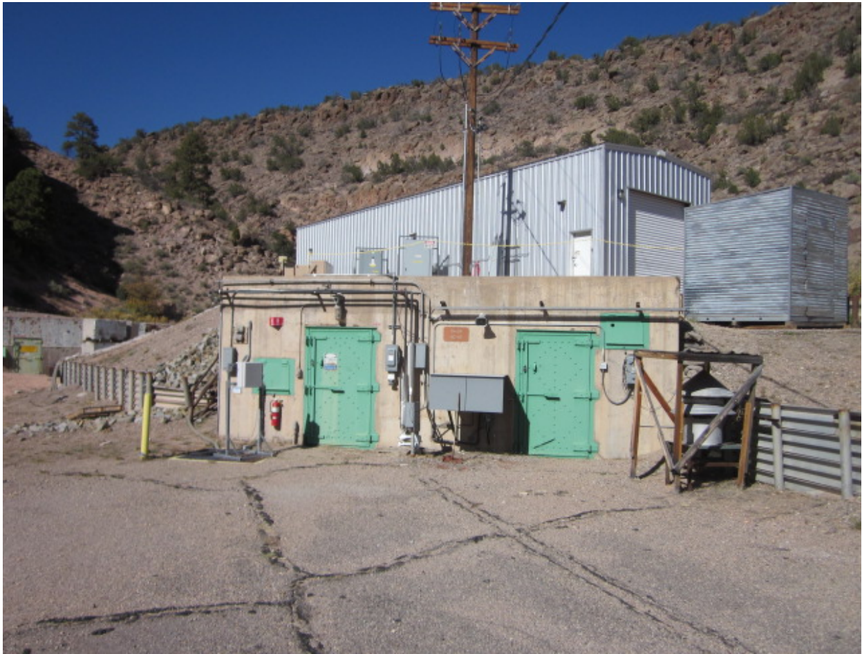
TA-39-57, Process Code X01, Open Detonation Unit
