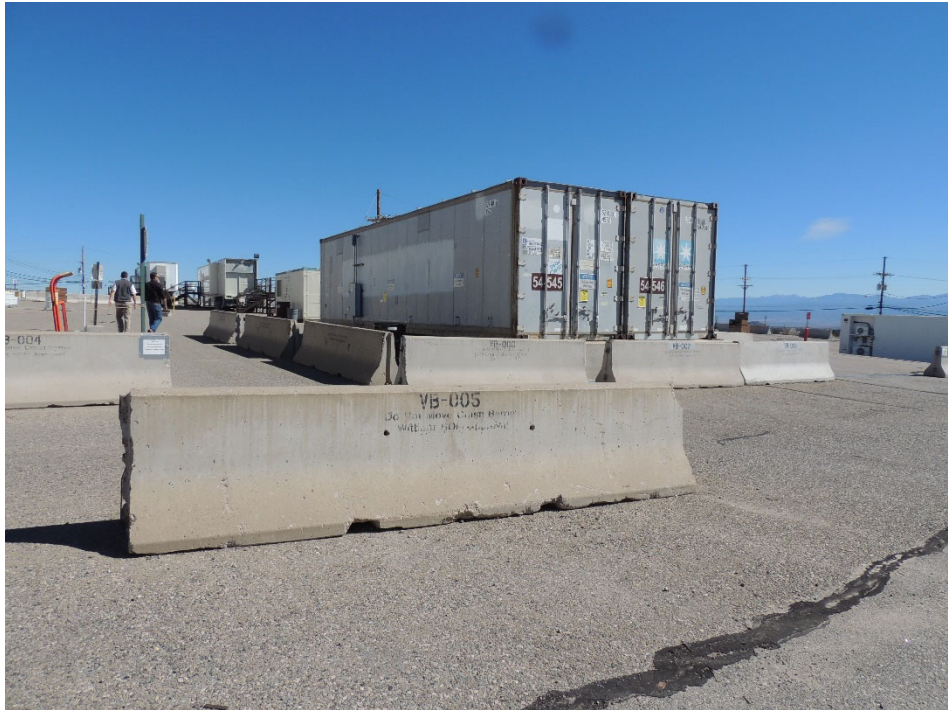
TA-54, Area G, Pad No. 10 Process Code S01, Container Storage Process Code T04, Other Treatment
