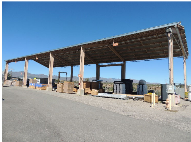
TA-54-35, TA-54-36 and TA-54-58, Area L, Process Code S01, Container Storage Units Process Code T04, Other Treatment
