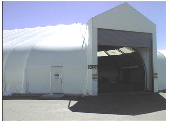
TA-54-230, Area G, Pad No. 9 Storage Dome Process Code S01, Container Storage Process Code T04, Other Treatment
