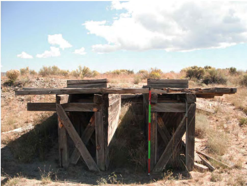
Photo 18-Looking east at LoadPly-1.
