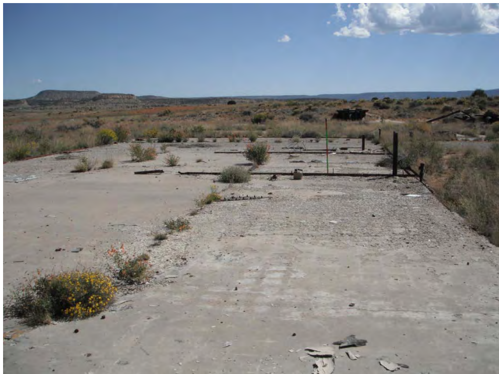
Photo 12-Looking east at StructPly-1.
