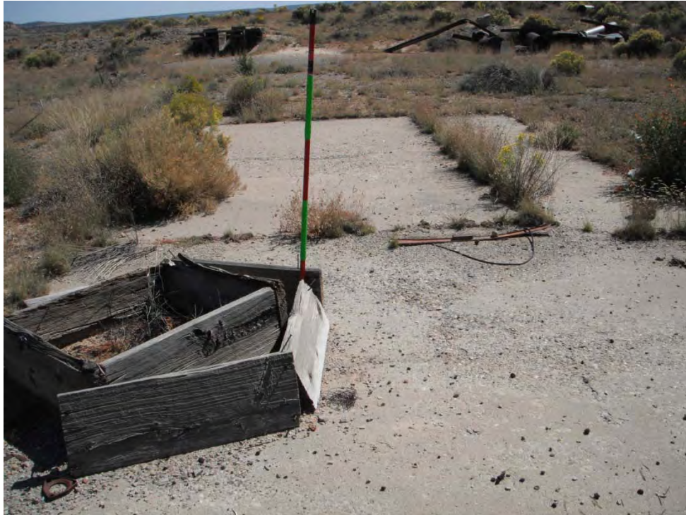
Photo 15-Looking east at StructPly-3.
