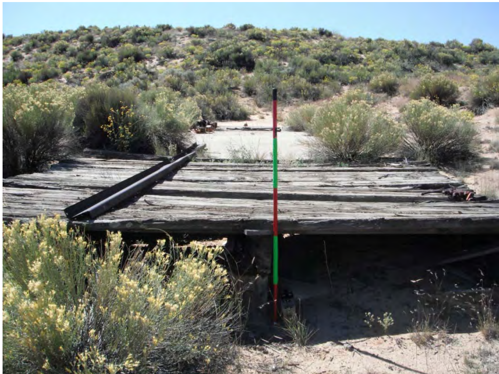
Photo 14-Looking south at StructPly-2.
